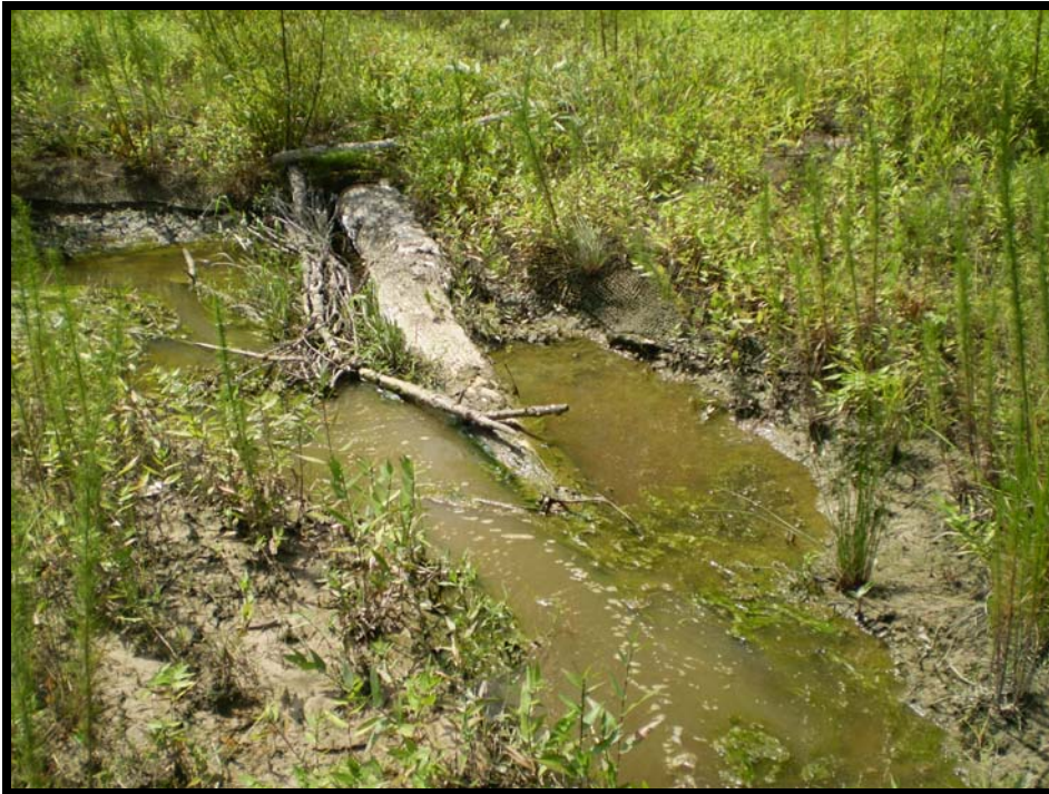
SPA8 – Erosion behind log vane @ station 74+50 (R3)
