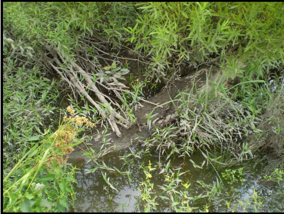
SPA3 – Erosion behind log vane @ station 33+75 (R2)
