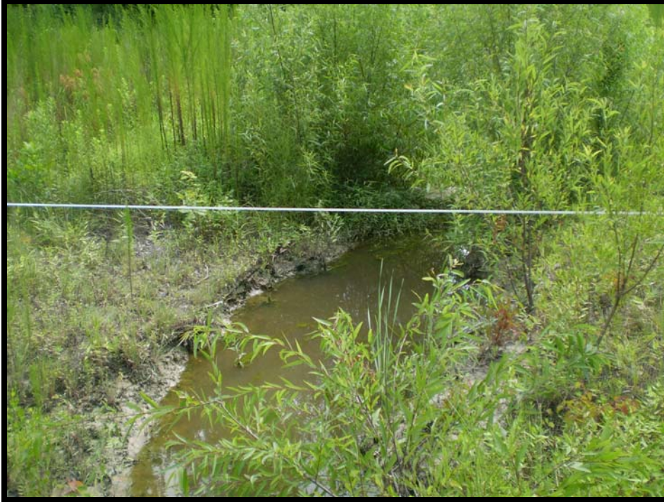
SPA9/SPA10 – Riffle downcut, erosion around rock weir @ station 74+90 (R3)
