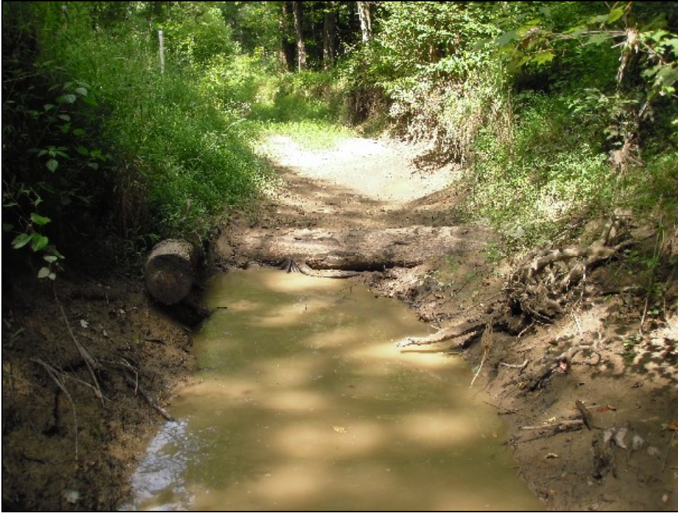
Reach 4 bedded log structure and woody debris, functional and stable.
