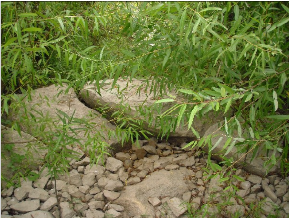
Stream Observation Area #4 – STA 75+00. Flow piping around header rock due to improper installation resulting in approximate one foot of bed loss.
