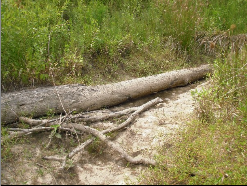
Stream Observation Area #3 – STA 74+50. Minor erosion behind log vane on right bank.
