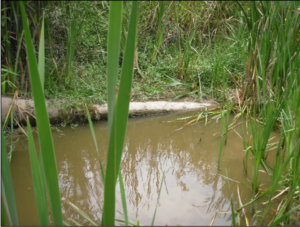
Reach 2 log vane, functional and stable.
