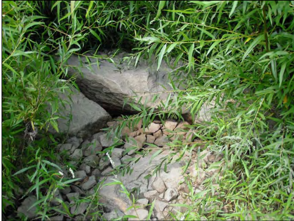
SOA #3 - Station 75+00, stable but non- functional rock grade control
