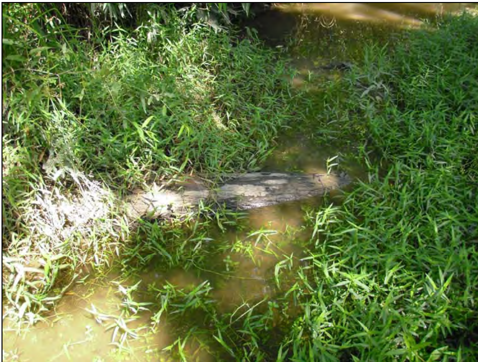
Station 69+60, stable and functional log vane
