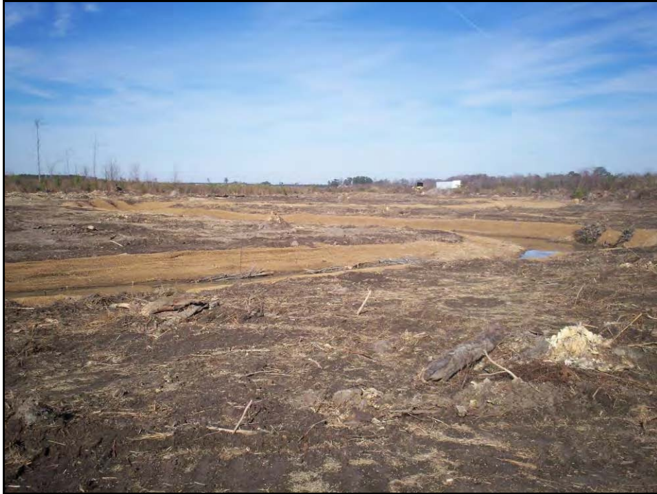
Reach 2 during construction phase.
