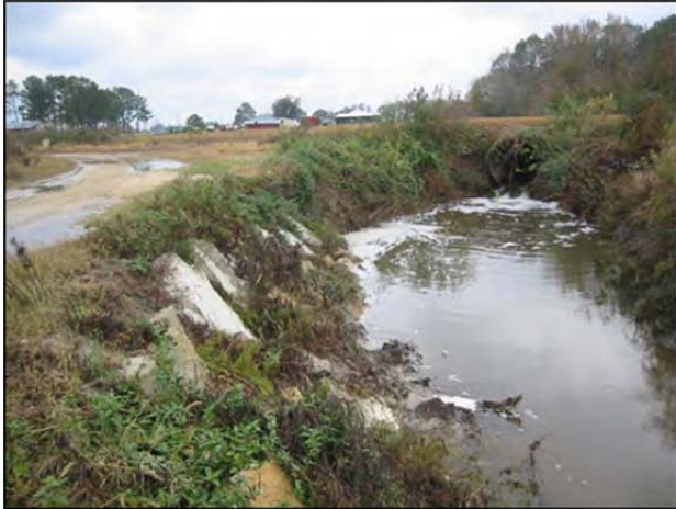
Upstream culvert, Reach 1 at Brown School Road during pre-construction phase.
