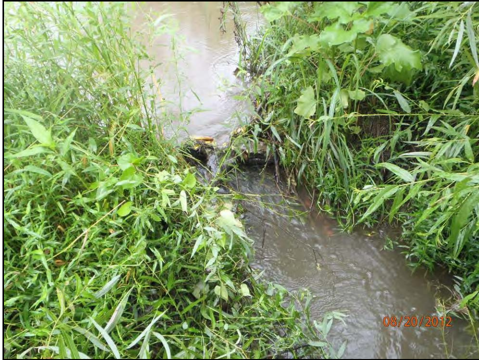
SOA #1 - Station 1+40, beaver dam in channel
