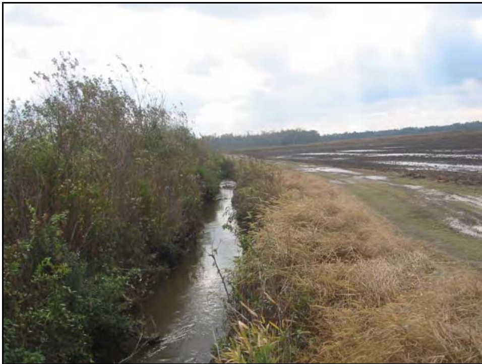
Reach 1 and 2 looking downstream during pre-construction phase.
