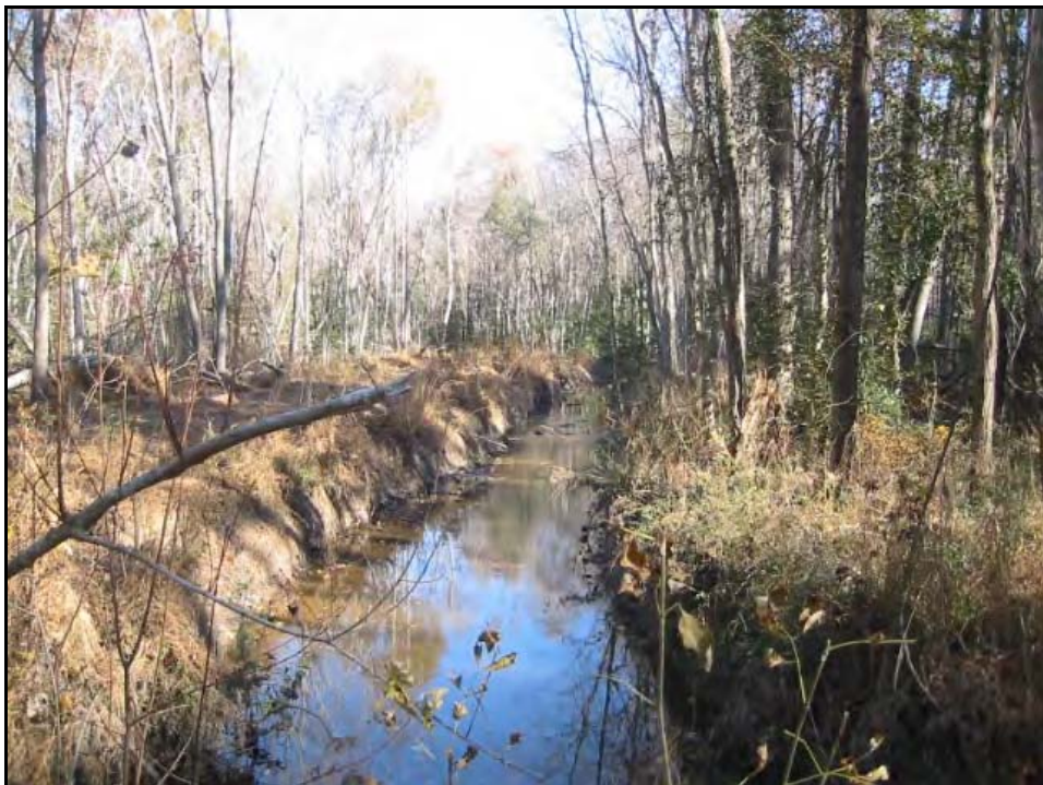
Reach 4 looking upstream during pre-construction phase.
