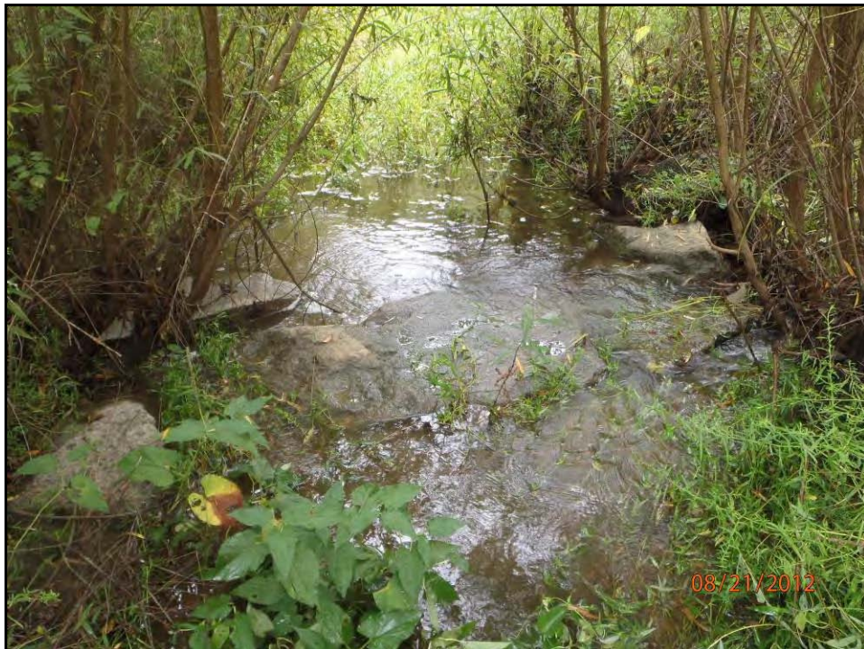
Station 75+00, Rock vane performing at bankfull conditions
