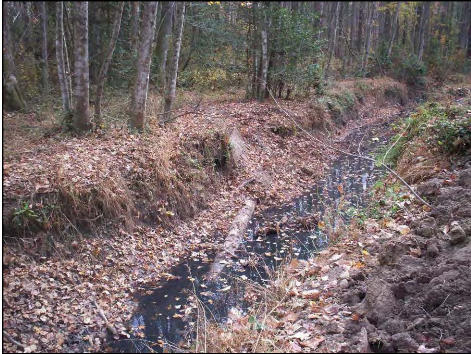
Reach 4 – Log vane installation during construction phase.
