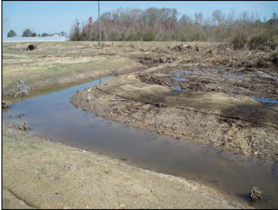
Reach 1 during construction phase.
