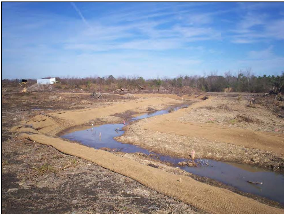
Reach 3 during construction phase.
