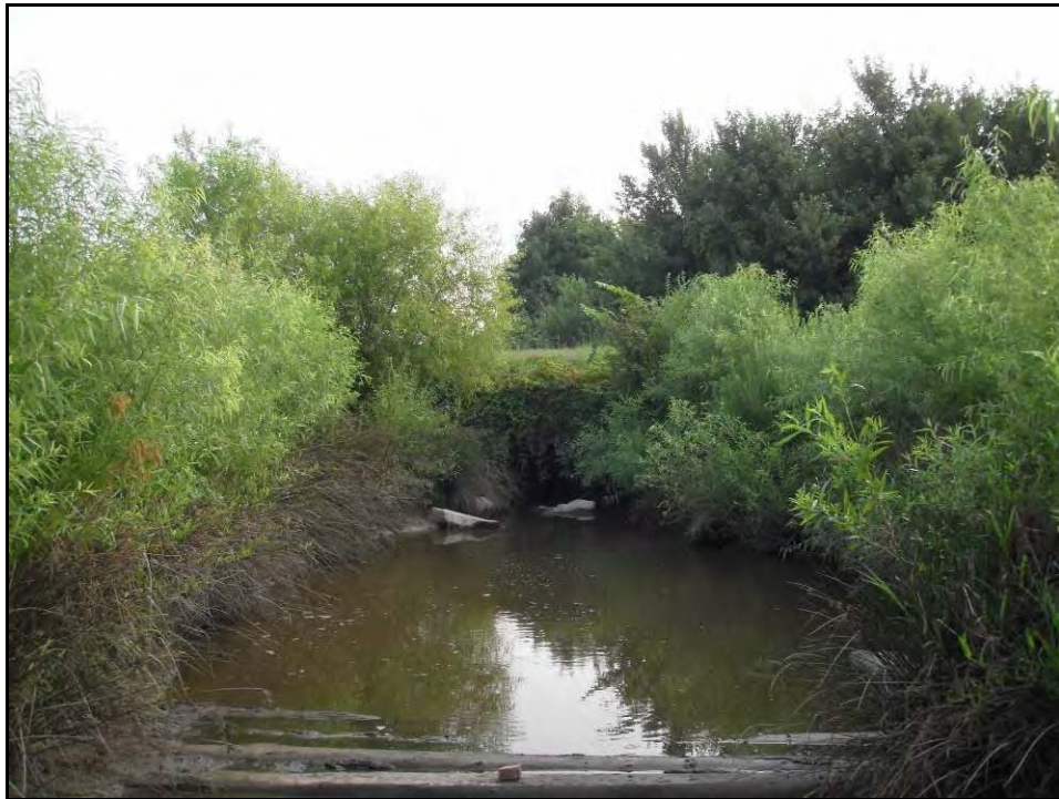
Upstream culvert, Reach 1 at Brown School Road during monitoring phase.
