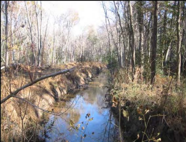
Reach 4 looking upstream during pre-construction phase.
