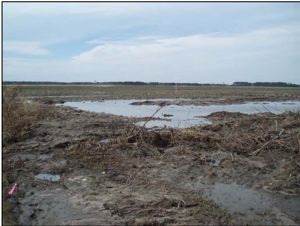
Wetland Restoration Area during construction phase.
