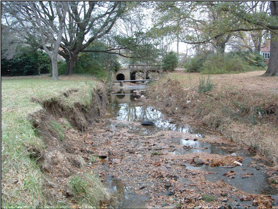
Upstream Project limits. (East Forest Hills Drive culvert/pipe, looking upstream.)
