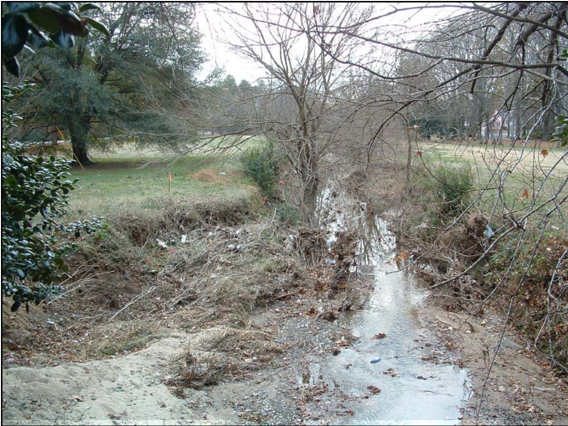
Degraded section downstream of E. Forest Hills Dr. crossing. (Sta. 30+50, looking downstream.)
