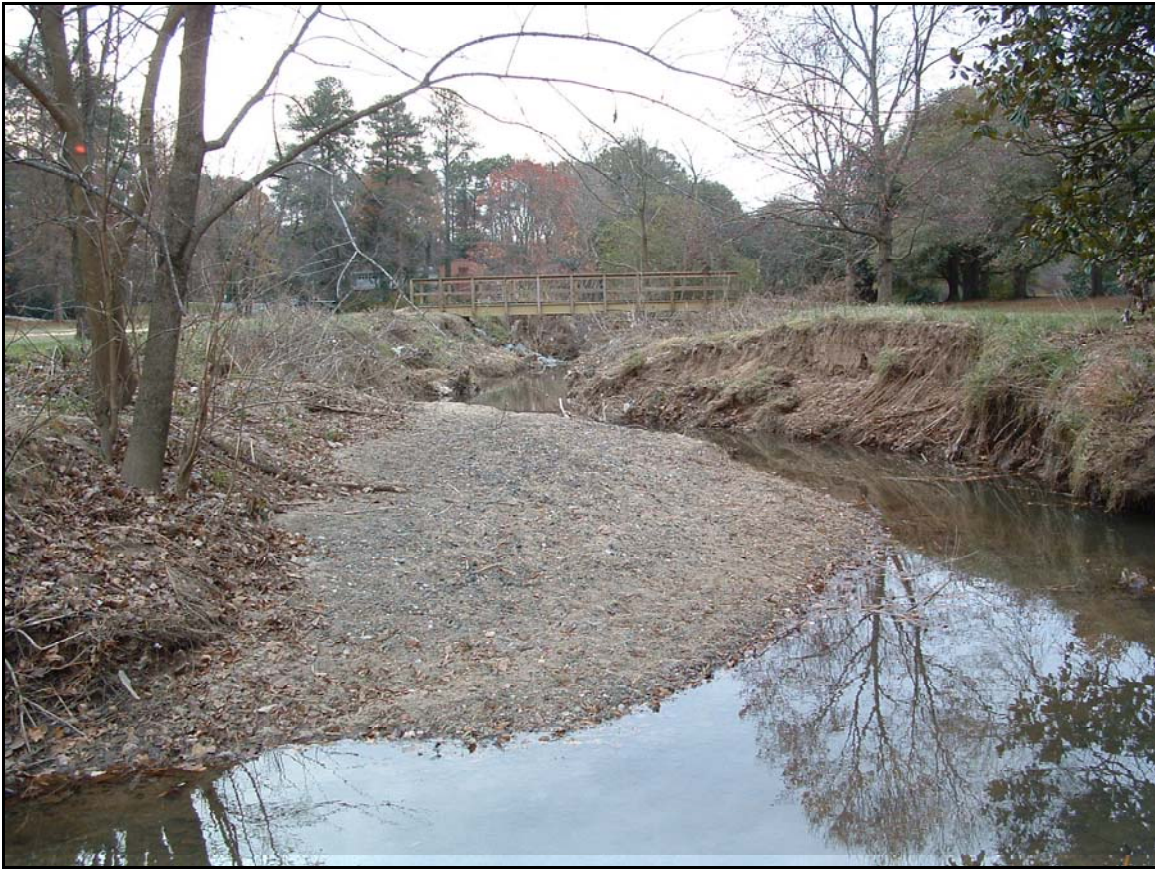
Existing steel/wood pedestrian bridge, to remain. (Sta. 38+40, looking downstream.)
