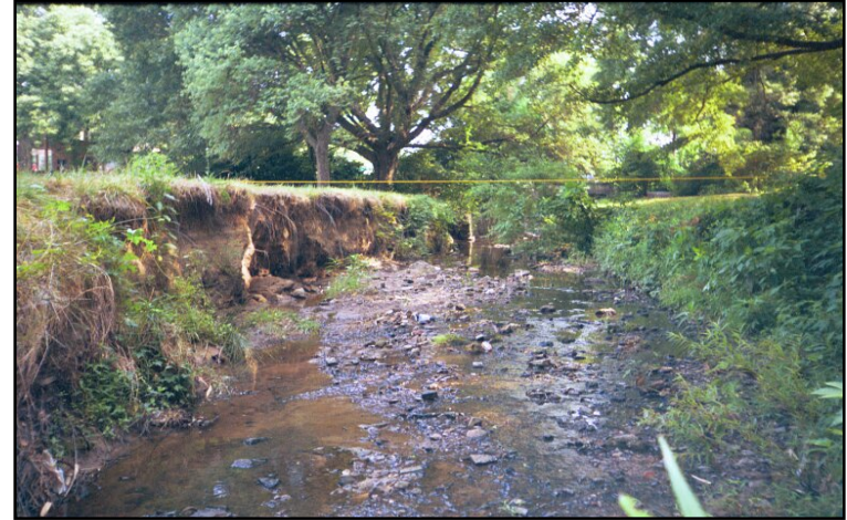
View looking upstream
