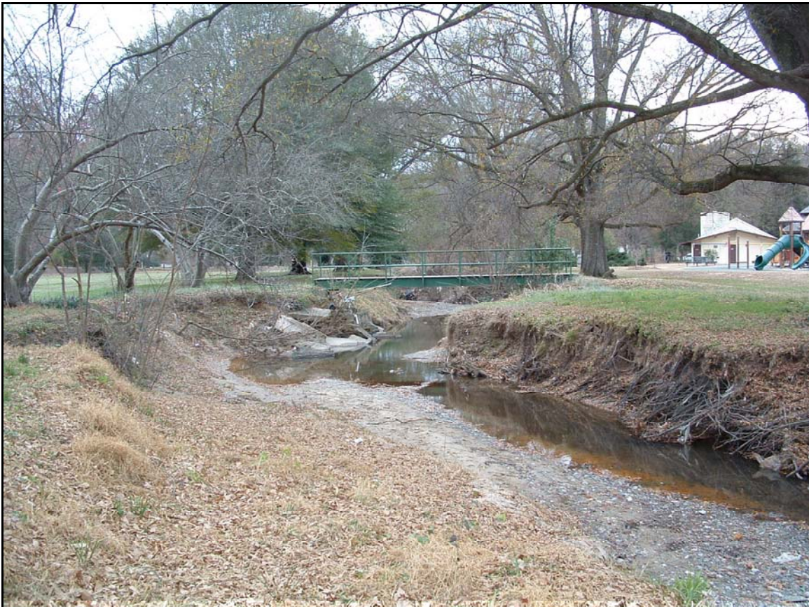
Existing concrete pedestrian bridge, to be removed. (Sta. 24+90, looking downstream.)
