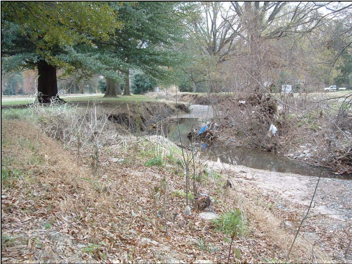
Typical section with eroding banks and developing lateral bars. (Sta. 23+00, looking downstream.)
