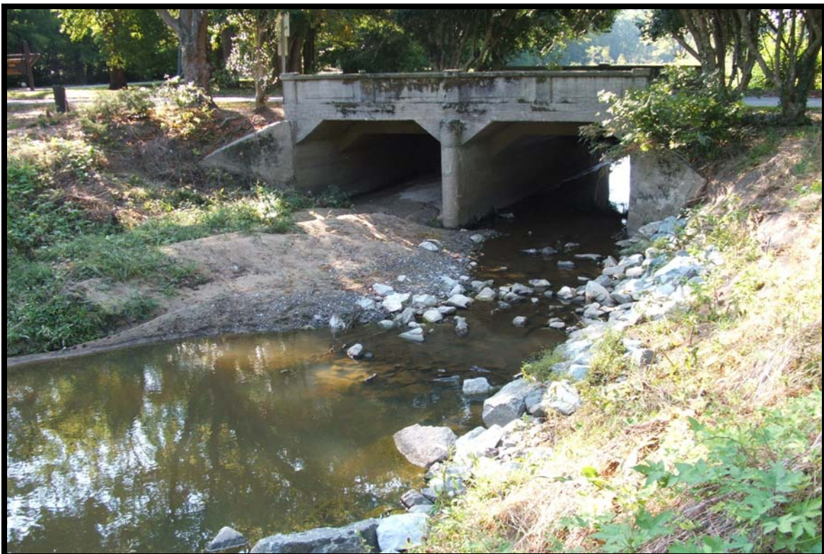
PRP 10 – Looking downstream.
