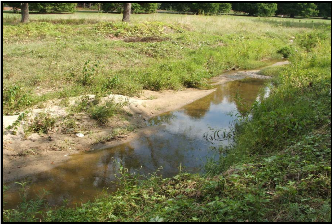
PRP 13 – Looking downstream.
