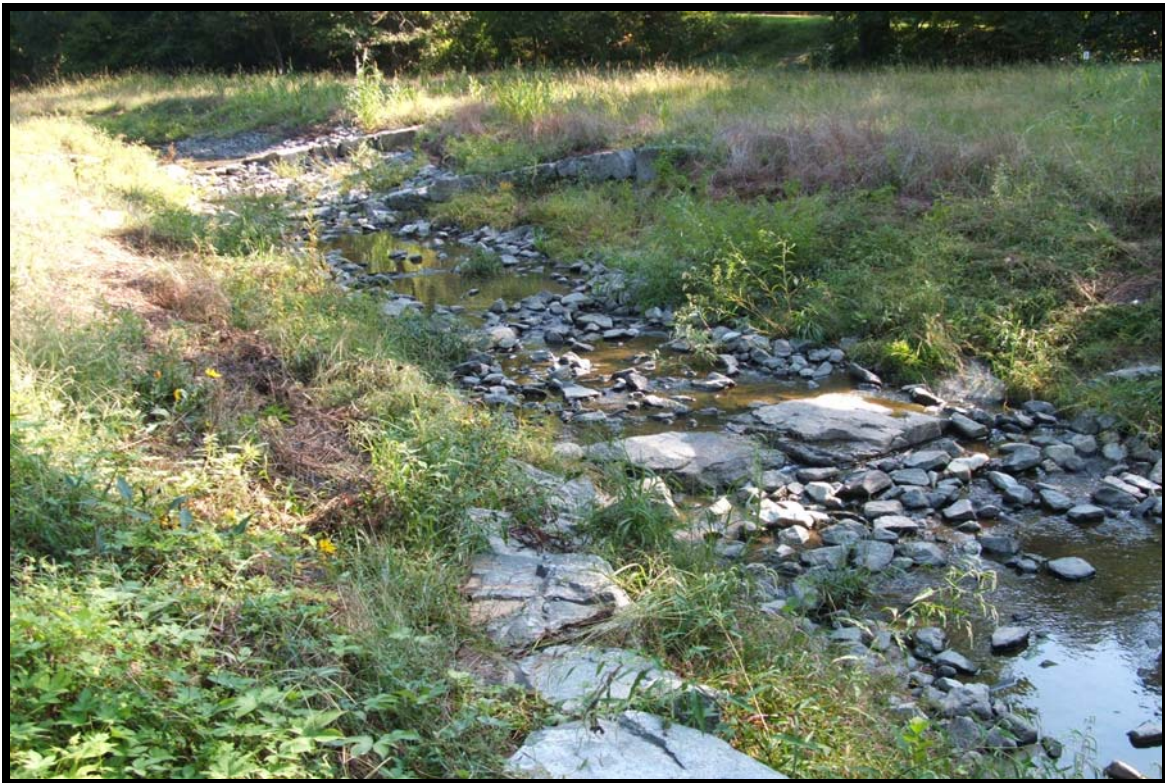
PRP 10 – Looking upstream. Note the stone from stream repair.
