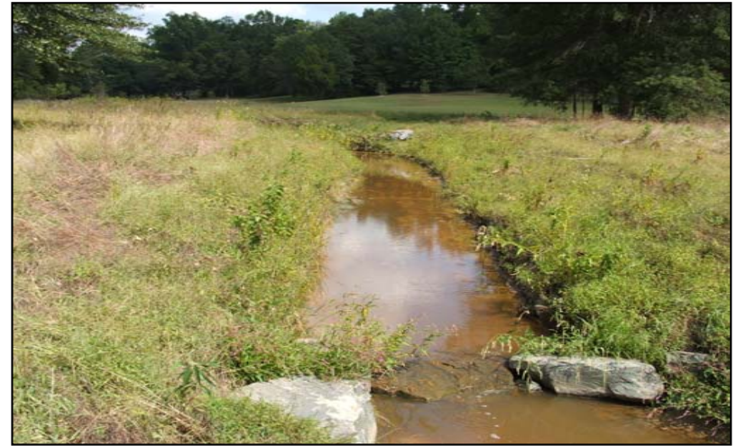
View of cross-section #1 looking upstream
