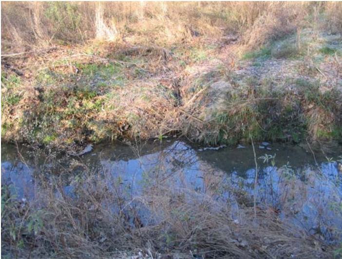
PP #3 – Ditch Entering Stream (11/20/06)
