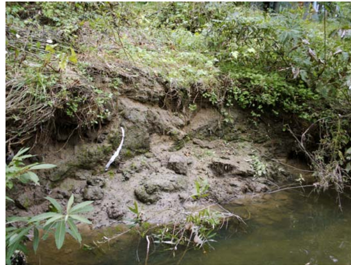
SP3. Bank undercut/slump
