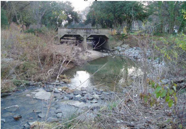
PP #10 – Looking Downstream (11/20/06)
