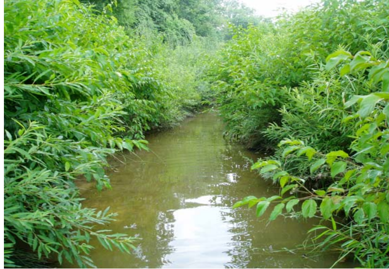
PP #7 – Looking Downstream (07/16/07)
