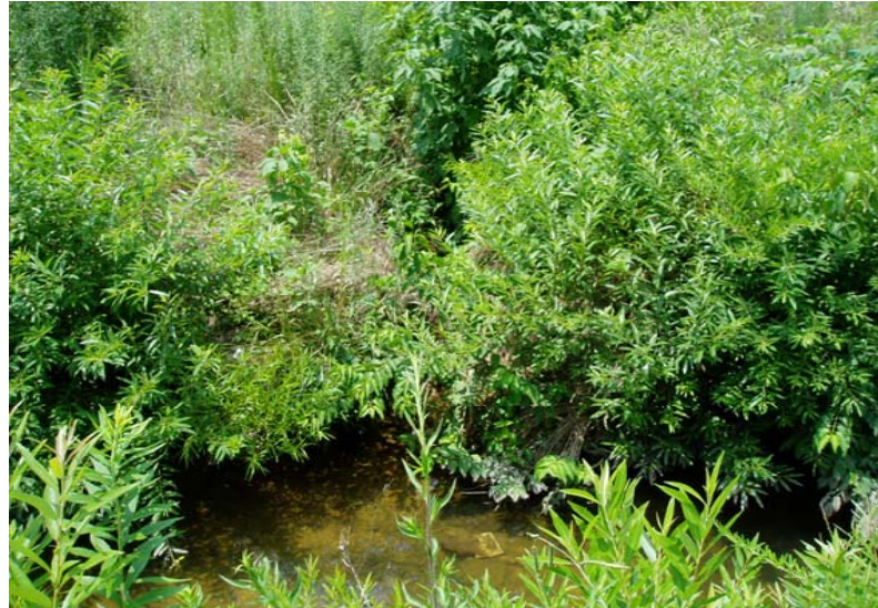
PP #3 – Ditch Entering Stream (07/16/07)
