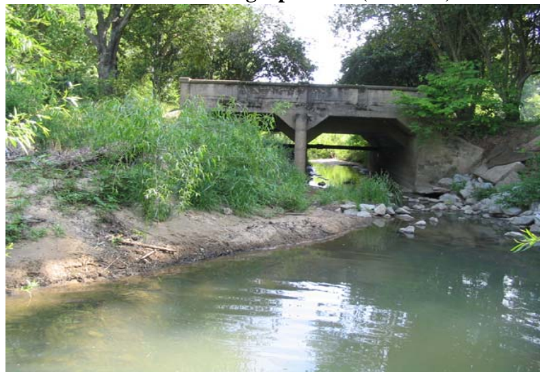
PP #10 – Looking Downstream (05/06/08)
