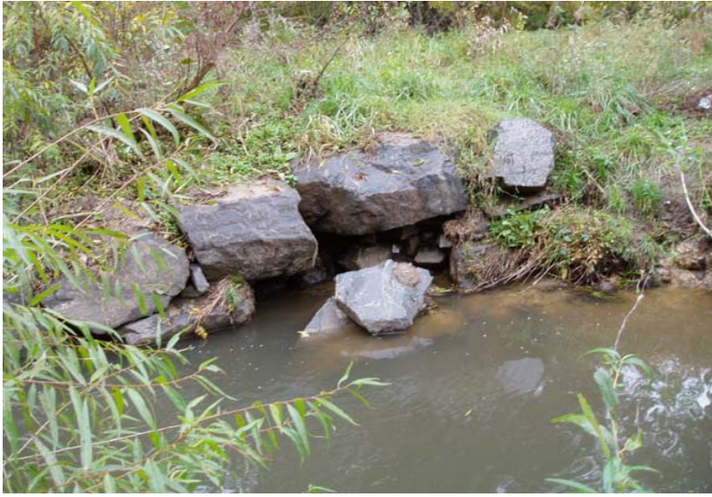
SP5-Boulder failure (10/28/2008)
