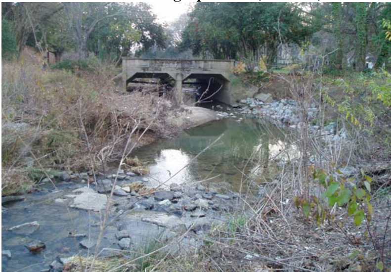
PP #10 – Looking Downstream (11/20/06)
