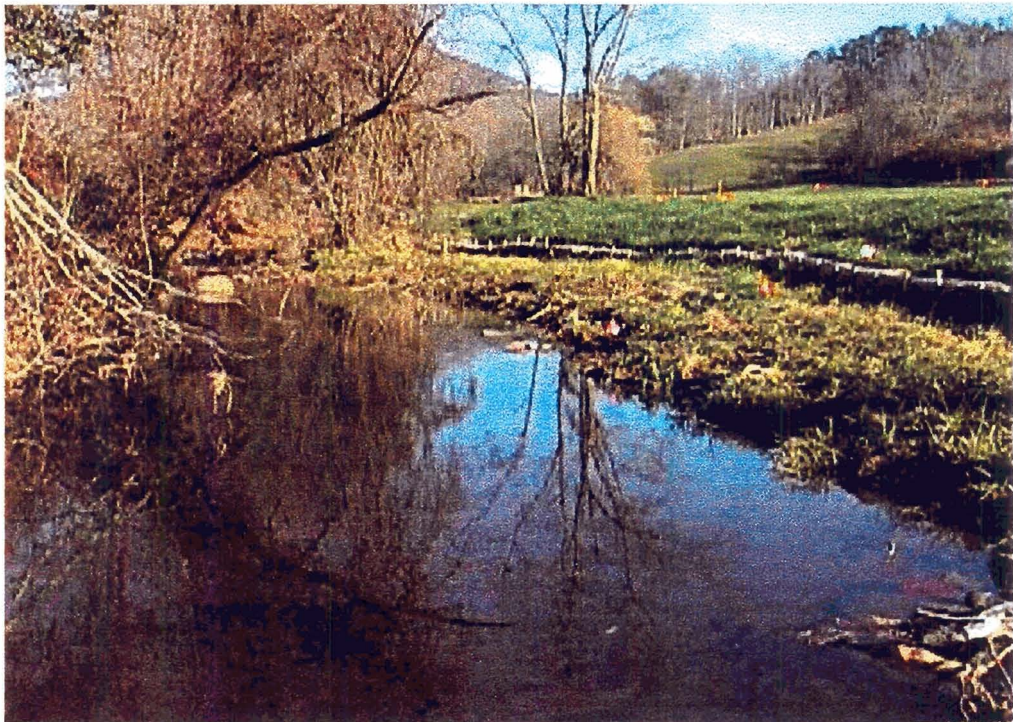
Upstream photo along lower end of site, showing the same location before and after construction. Note the willow tree and walnut trees (center top of photos) for reference. Vertical, eroding stream banks have been sloped and vegetated for greater stability.
