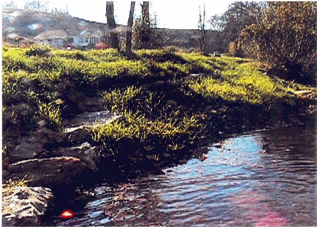
Photo downstream at same location before and after construction. Photos show the change in stream bank profile, stabilization with vegetation and erosion control materials and a rock vane constructed to direct flow toward the thalweg and reduce pressure on the near bank region.
