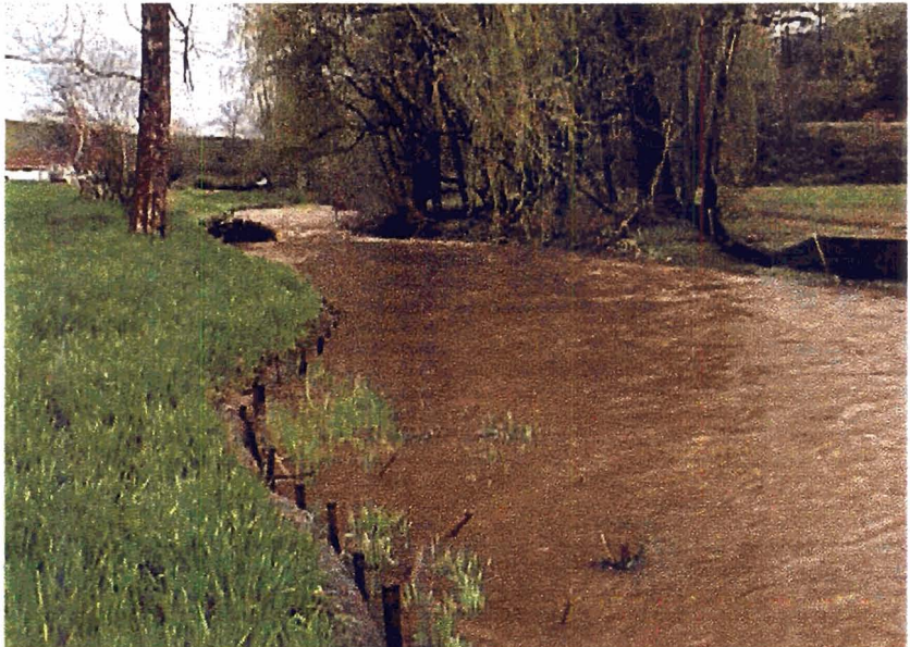
Downstream photo at same point before and after construction, showing sycamore for reference. Bottom photo shows same site during bankfull event.
