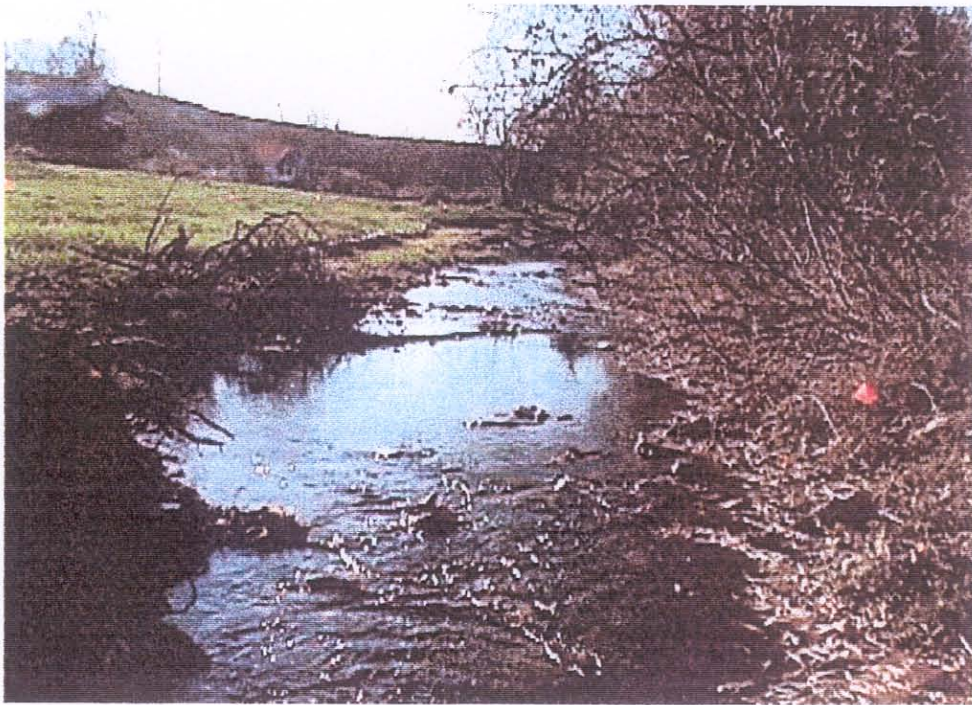
Downstream photo of same location showing lower rootwad revetment and banks before and after construction
