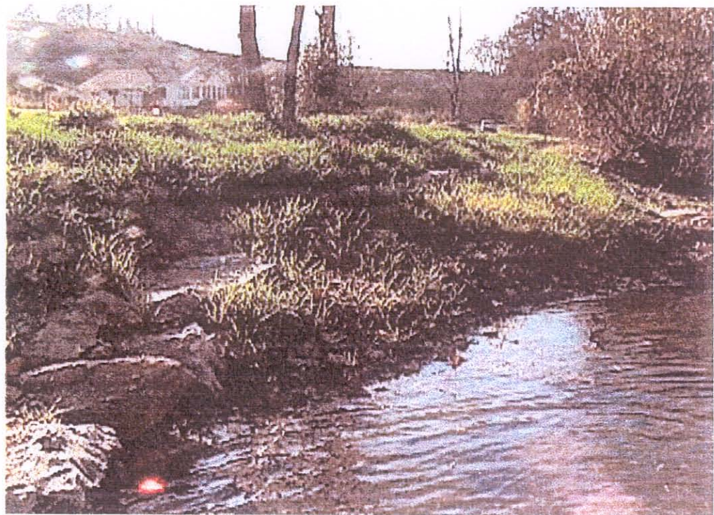
Photo downstream at same location before and after construction. Photos show the change in stream bank profile, stabilization with vegetation and erosion control materials and a rock vane constructed to direct flow toward the thalweg and reduce pressure on the near bank region.
