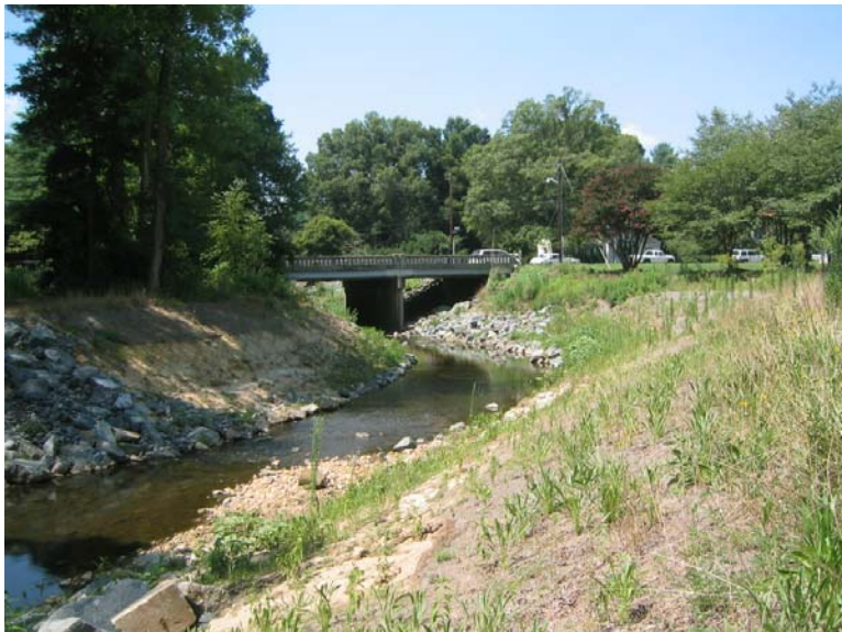
P23. Looking Downstream at the end of the project (Station 44+00)
