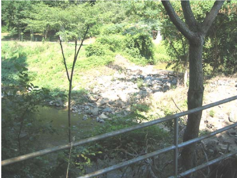
P12. Looking Downstream from Bridge (Station 22+80)
