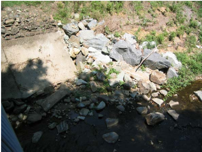
P19. Bridge Abutment Looking Upstream Right Bank (Station 36+40)
