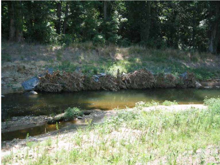
P21. XSC-9 Left Bank (Station 40+80)
