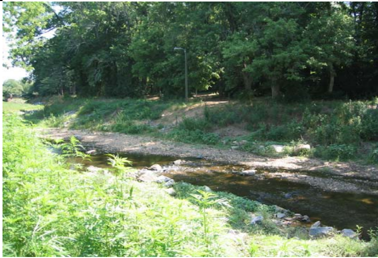
Photo of Cross-Section #5 - Looking Upstream
