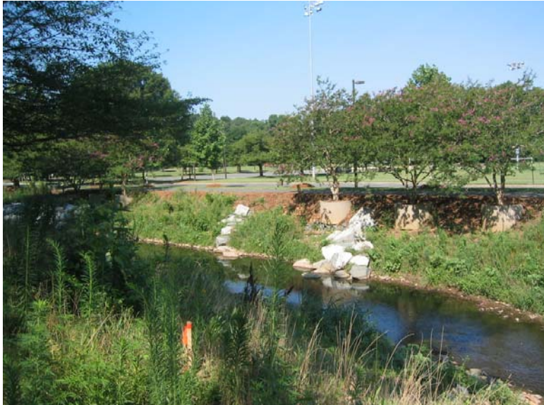
P6. XSC-3 Looking Downstream (Station 14+00)
