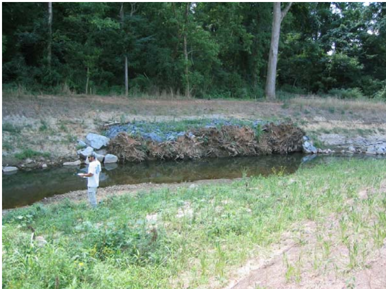
P20. XSC-9 Left Bank (Station 40+20)
