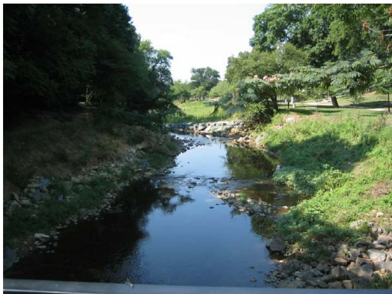
P11. Below XSC-4 Looking Downstream (Station 19+20)
