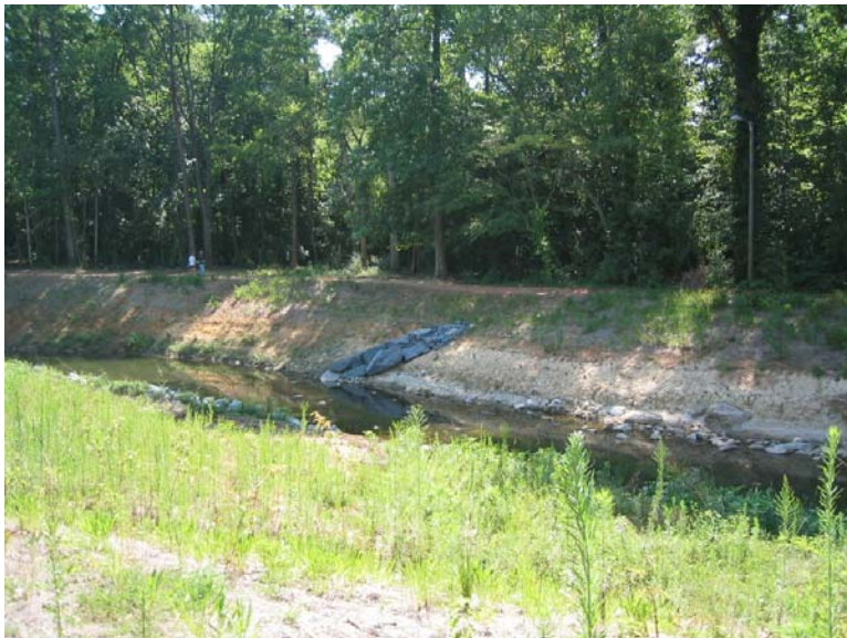
P14. XSC-6 Looking Upstream (Station 27+50)
