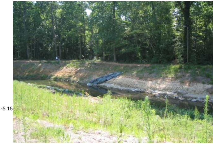
Photo of Cross-Section #6 - Looking Upstream
