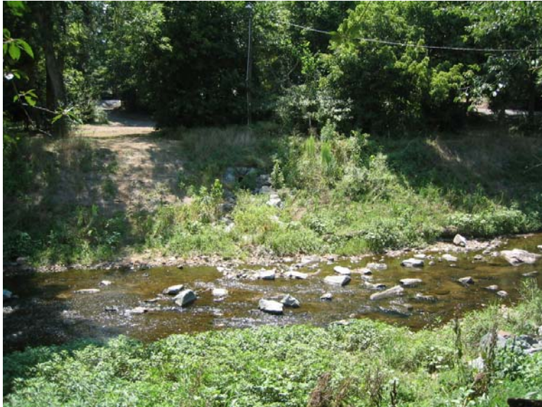
P18. XSC-8 Left Bank (Station 34+40)
