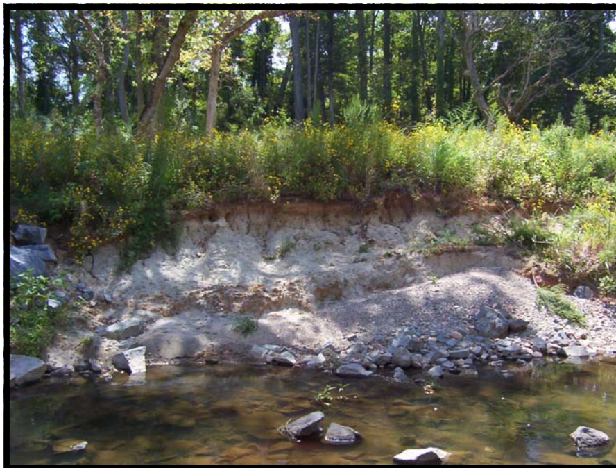
Photo 2—Typical Bank Scour
