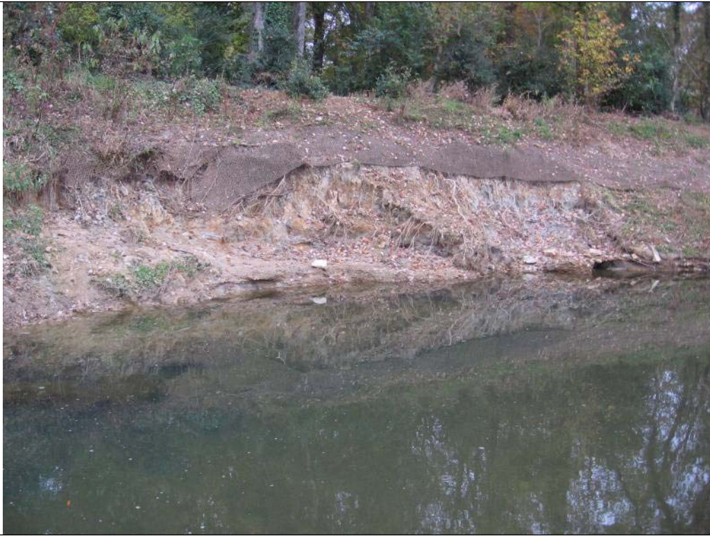
SP 7: Scour between root wads – possible displacement of root wads
