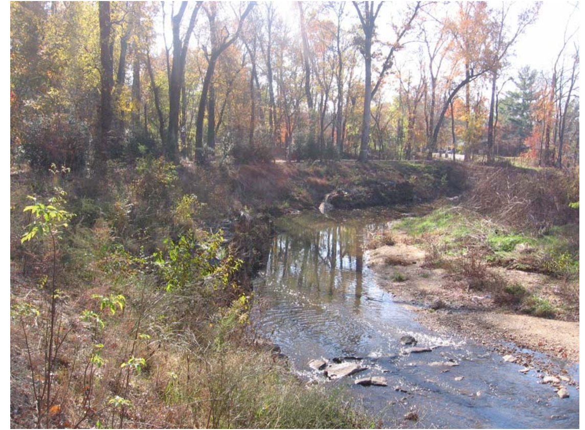
SP 6: Looking downstream at left bank, scour between root wads
