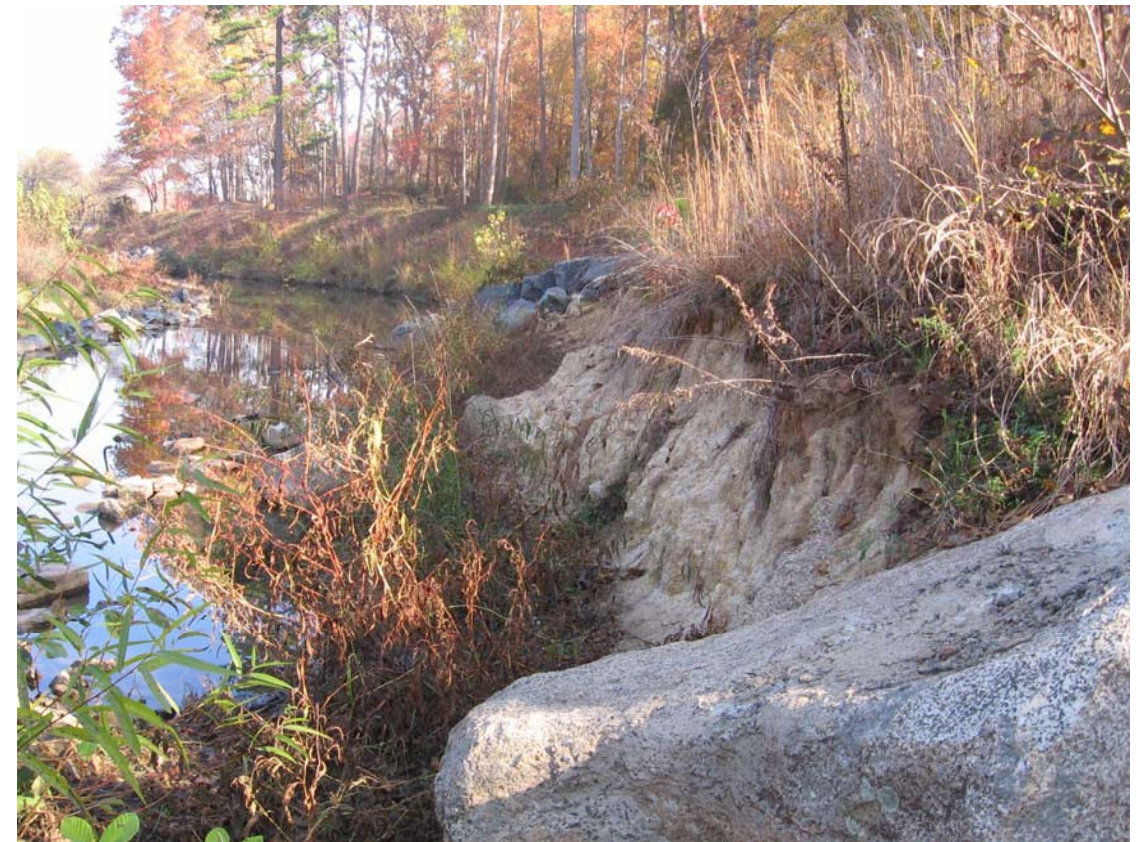
SP 4: Looking upstream at left bank, scour
