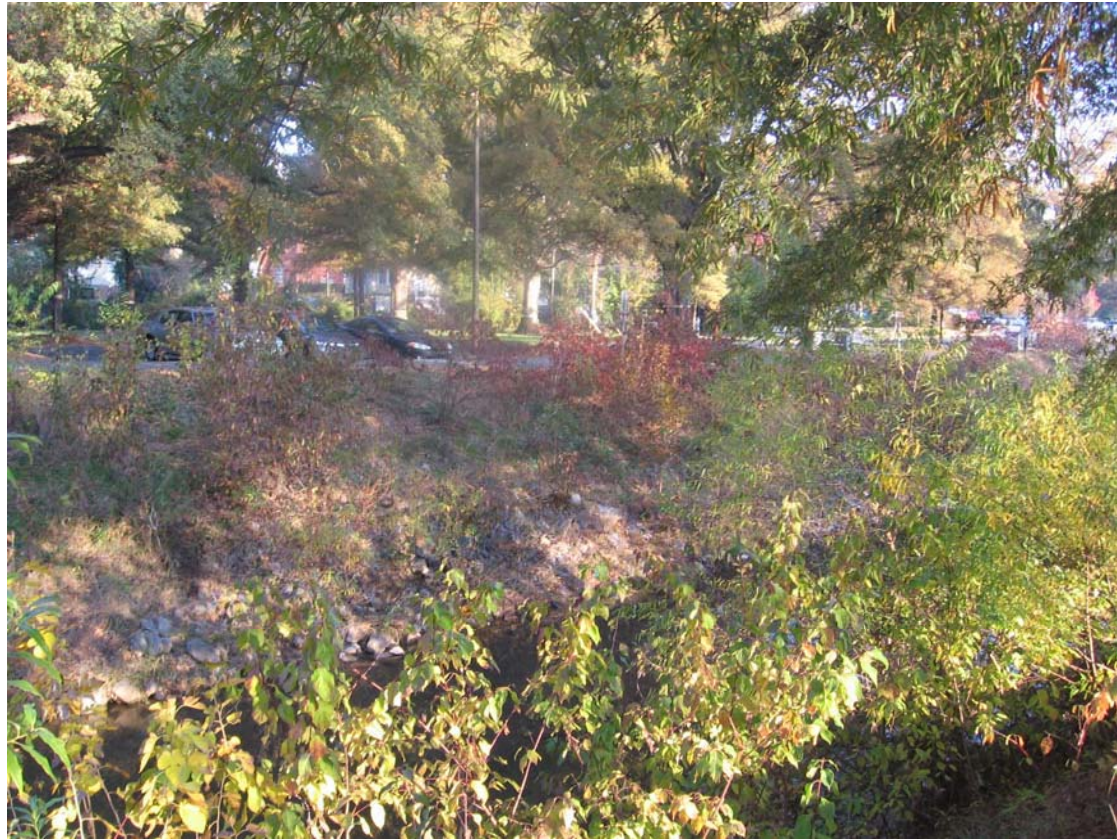
VP 1: Looking at right bank, bare bank
