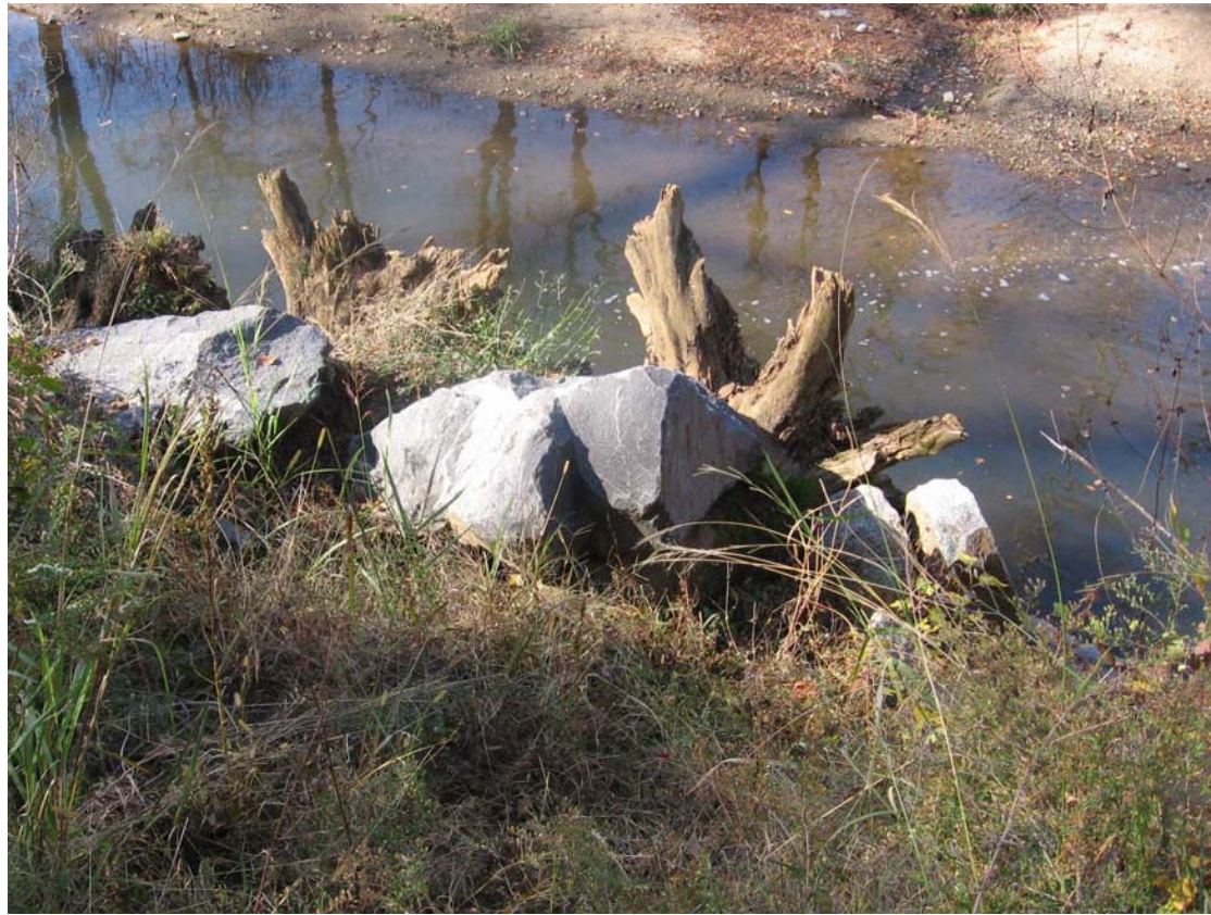
SP 7: Looking at left bank, root wads stabilized by boulders
