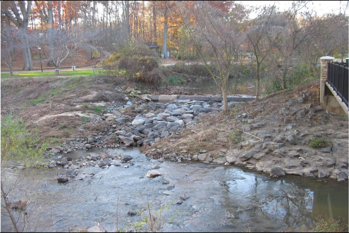
Permanent Photo PS12 Taken On: 11/14/2006
