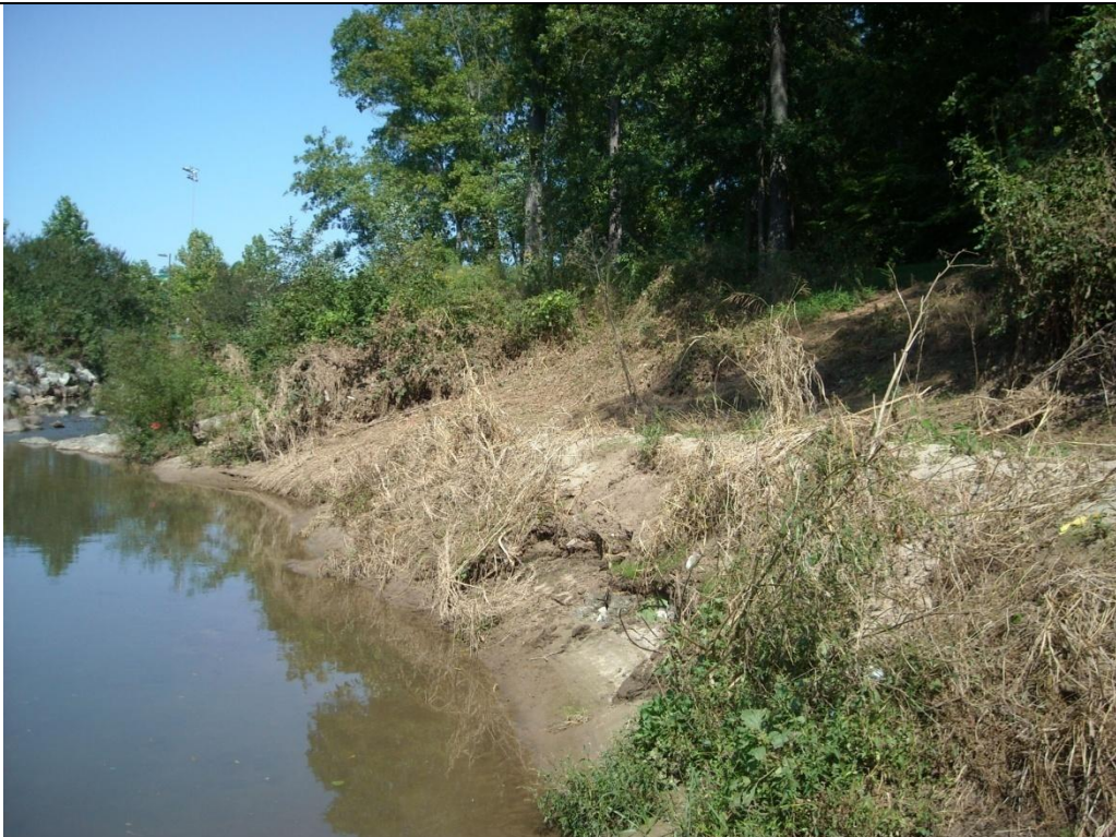
SP1: Bank erosion in area of limited woody vegetation Taken 9/24/2008
