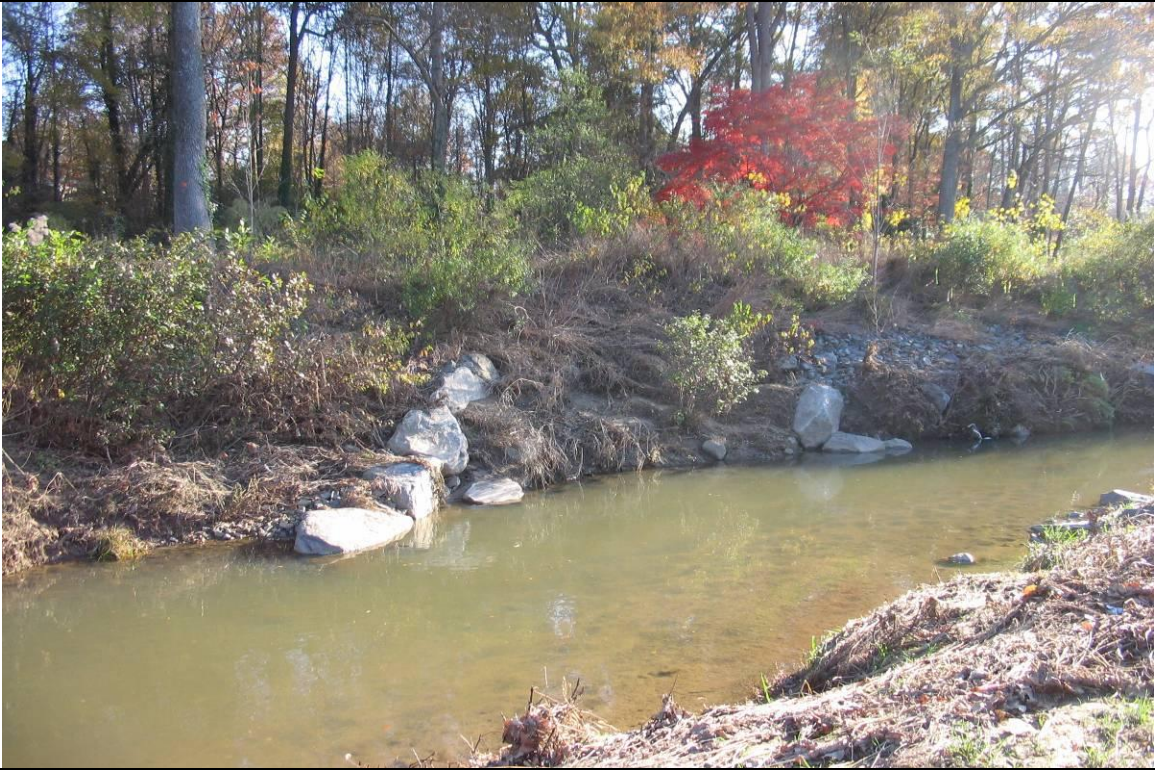
Permanent Photo PS03 Taken On: 11/14/2006
