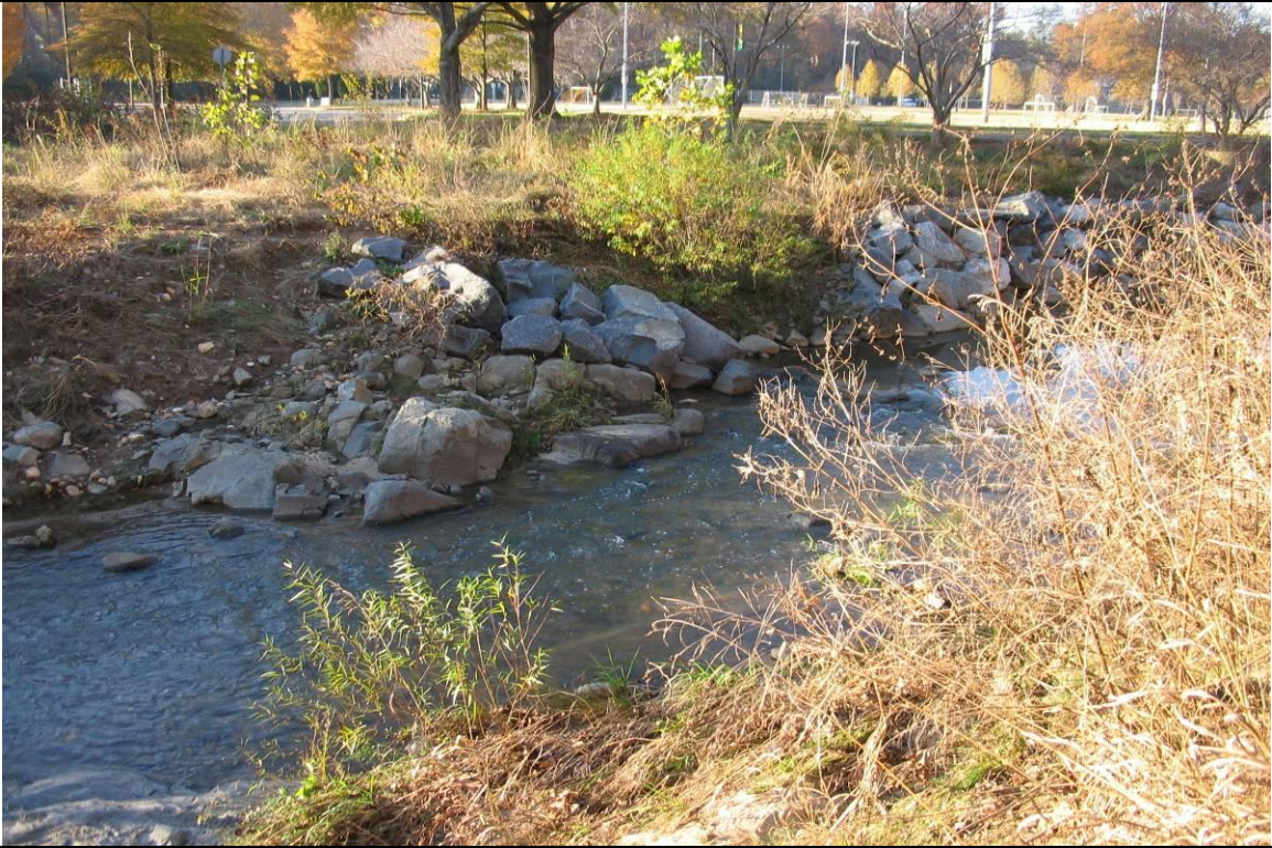
Permanent Photo PS09 Taken On: 11/14/2006
