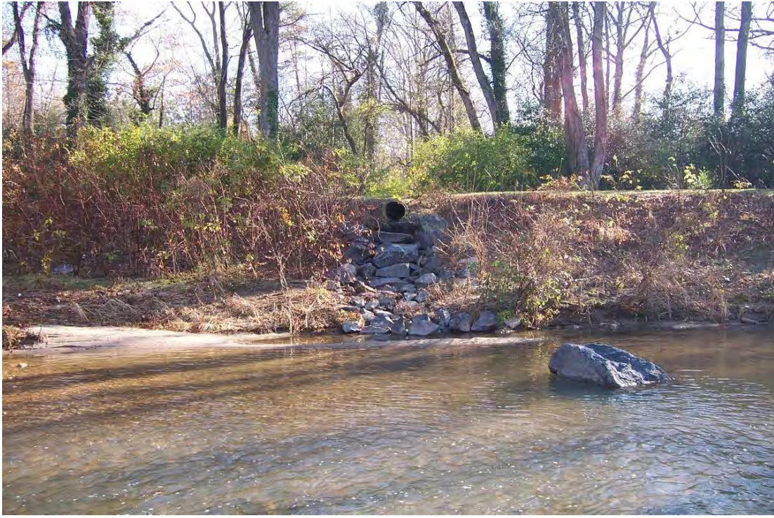
Permanent Photo PS16 Taken On: 11/14/2006
