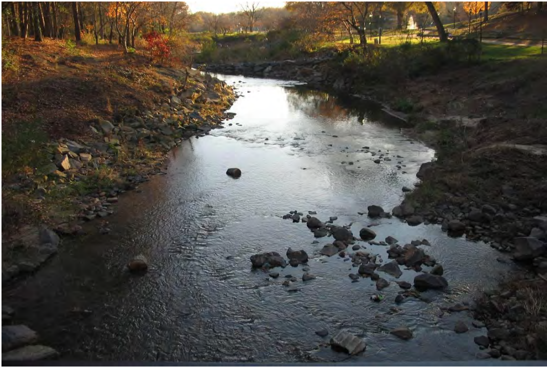
Permanent Photo PS11 Taken On: 11/14/2006
