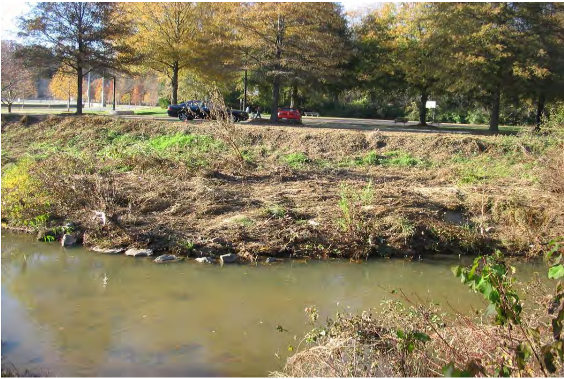
Permanent Photo PS02 Taken On: 11/14/2006
