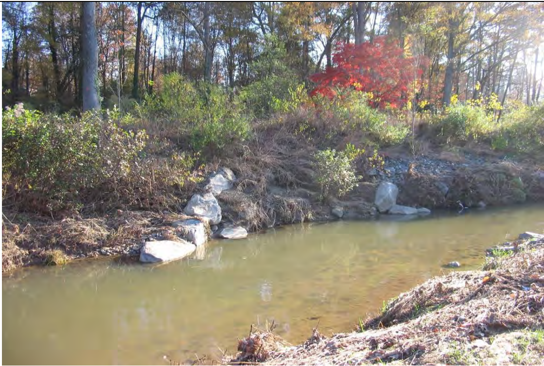
Permanent Photo PS03 Taken On: 11/14/2006
