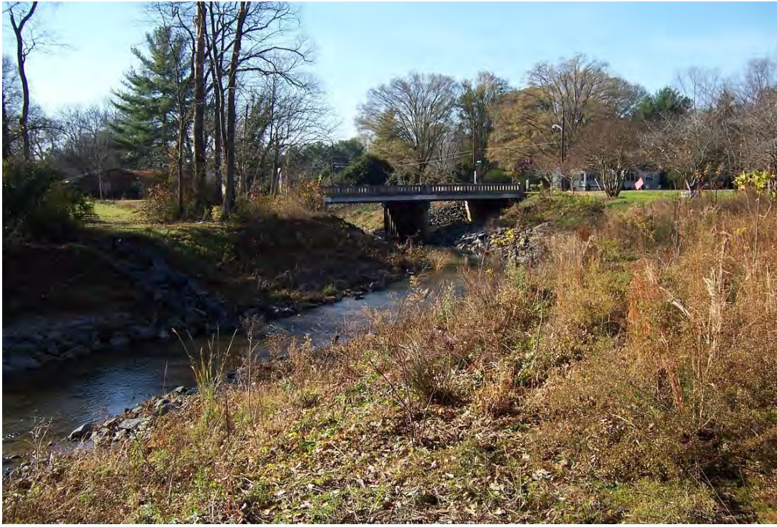
Permanent Photo PS23 Taken On: 11/14/2006
