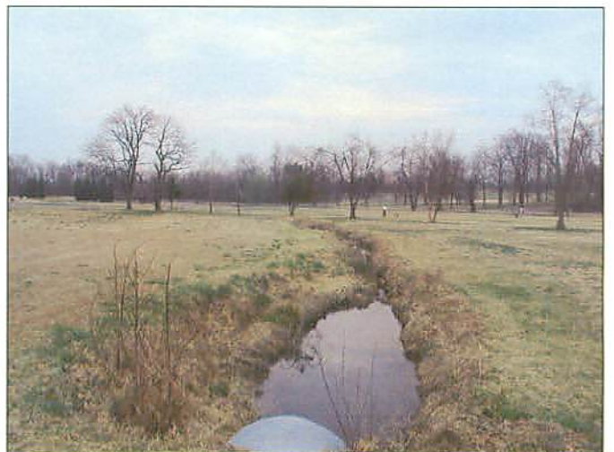
PP28 Reach 4 Looking Downstream
