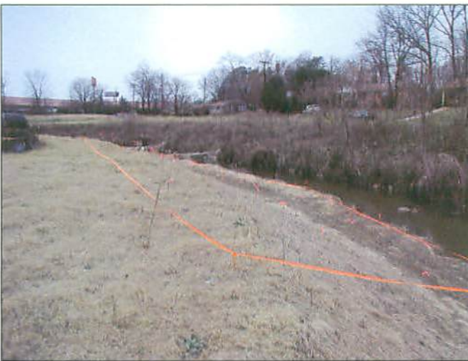
PP8B Forested Buffer Bareroot Vegetation Plot Looking Upstream From Top of Terrace at Station 18+00
