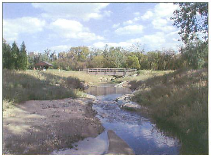
PP14 Reach 1E Towards Bridge 3
