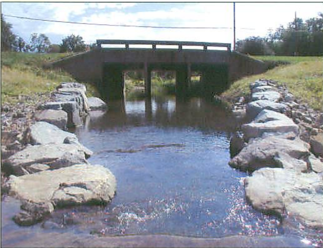
PP12 Reach 1A Cross Vane #1 & Vanstory Culvert
