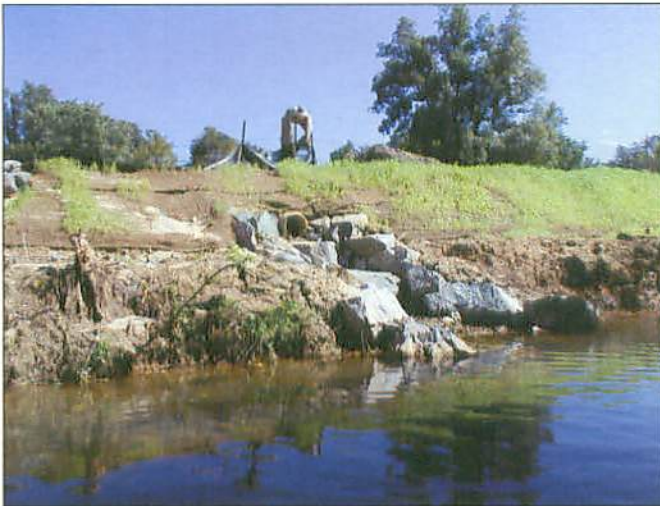
PP34C Reach 2 Step Pool #2 Before Repairs
