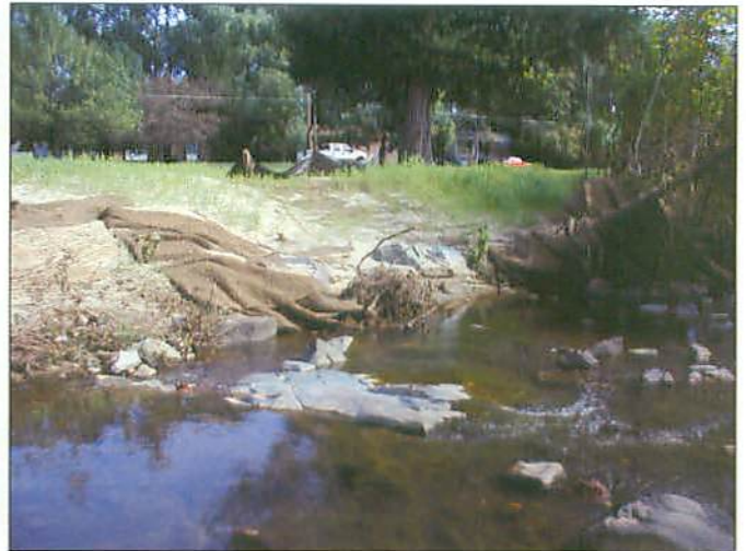
PP30C Reach 2 Rootwad #1 Before Repairs
