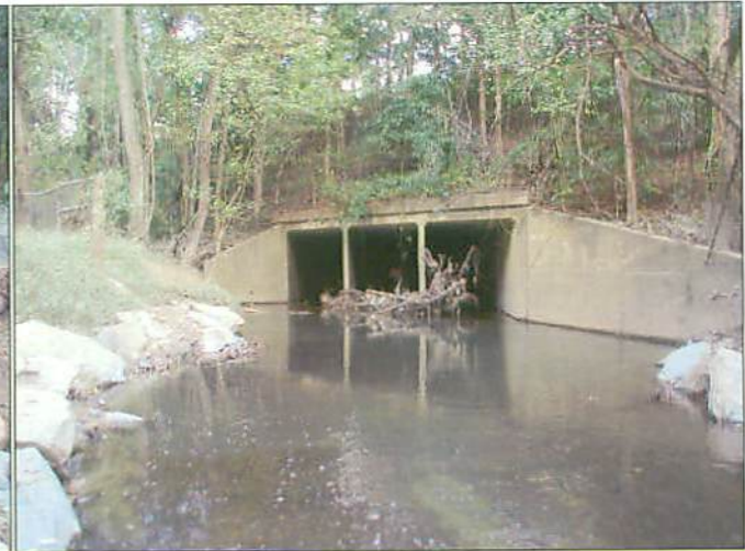
PP19 Reach 1F Project End
