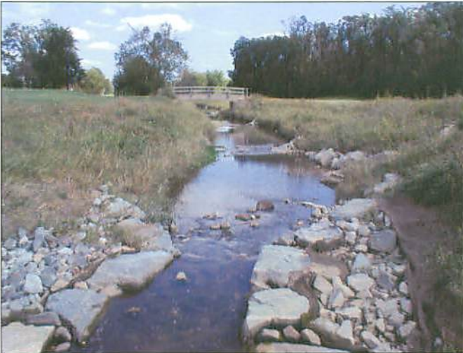
PP7 Reach 1B Towards Bridge 2
