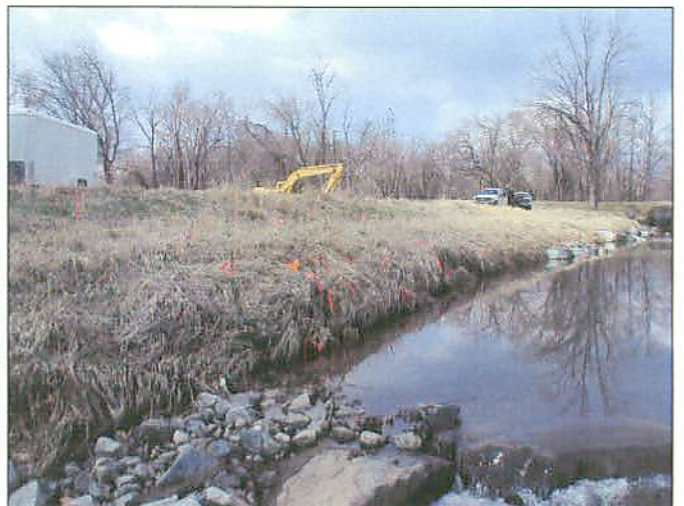
PP3B Reach 1A Forrested Buffer Bareroot/Livestake Plot Looking Upstream
