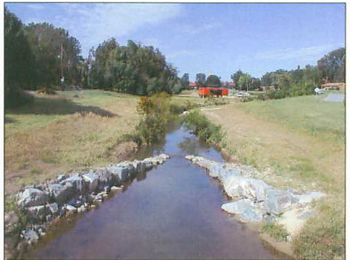
PP13 Reach 1A End (Upstream view)
