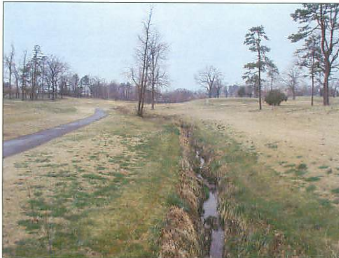
PP27A Reach 4 Looking Upstream
