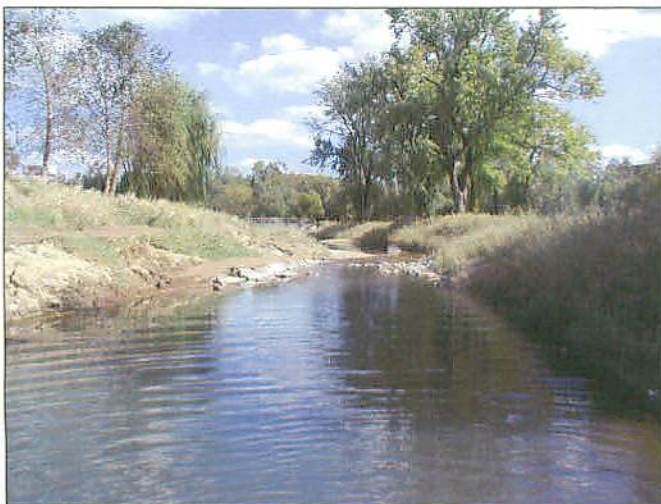
PP13 Reach 1D Constructed Riffle
