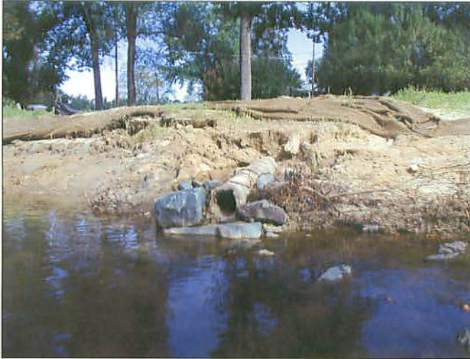
PP30B Reach 2 Step Pool #1 Before Repairs
