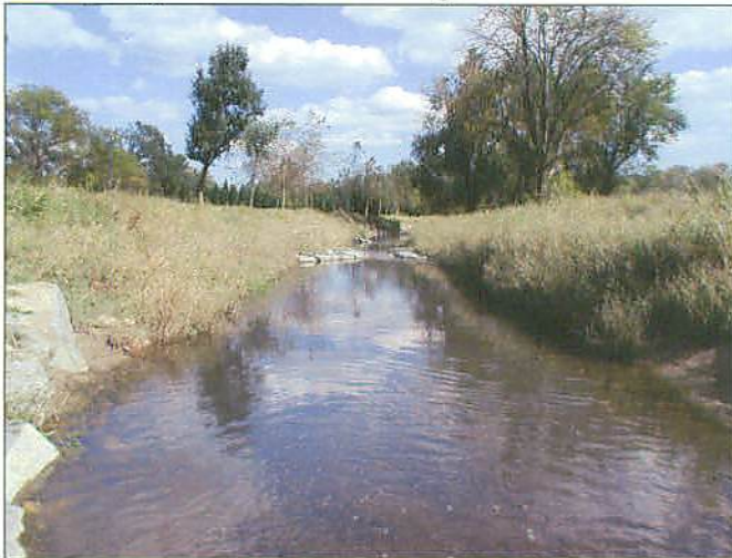
PP11 Reach 1D Double Wing Deflector #1
