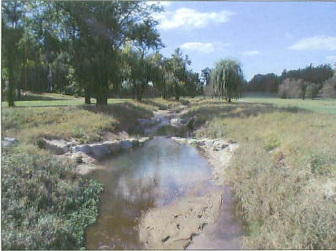
PP15A Reach 1E Looking Upstream
