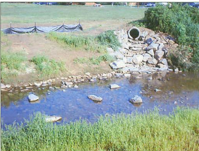
PP5 Reach 1A Constructed Riffle #1 & Step Pool #1
