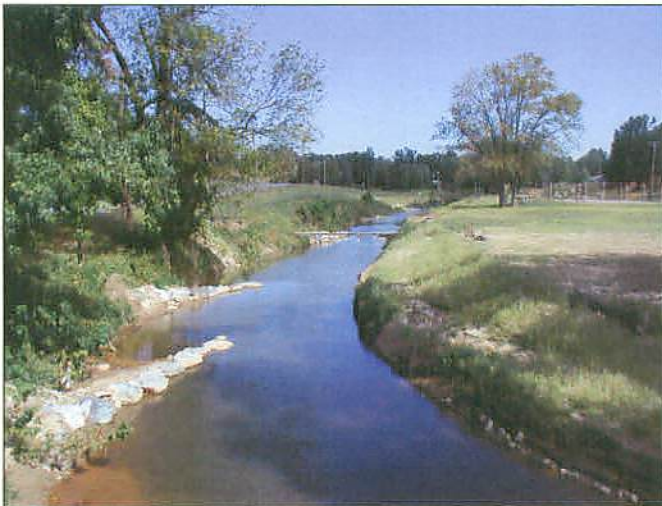
PP27 Reach 1B End (Upstream View)
