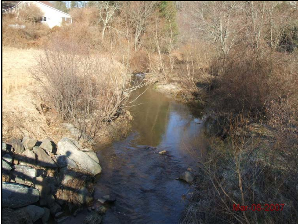
Glade Creek Pre-construction conditions looking upstream from Photo Station 5
