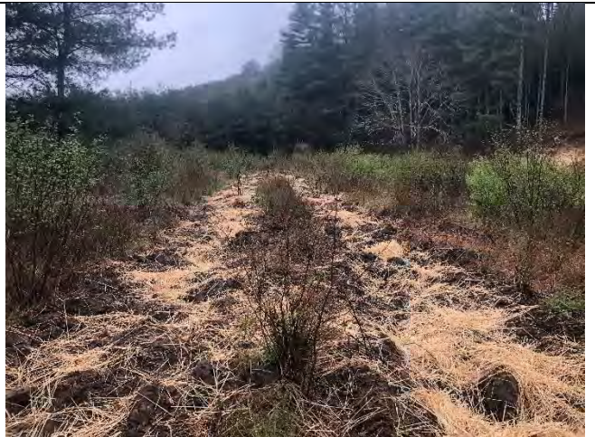
Construction access route stabilization
