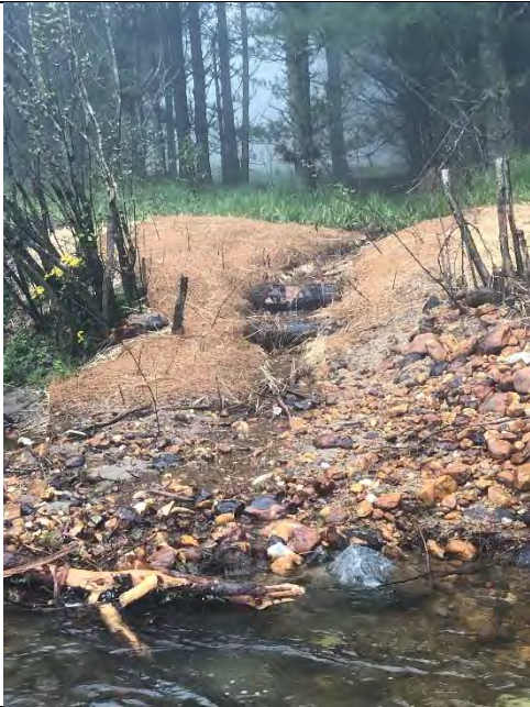
Wetland B outlet steps
