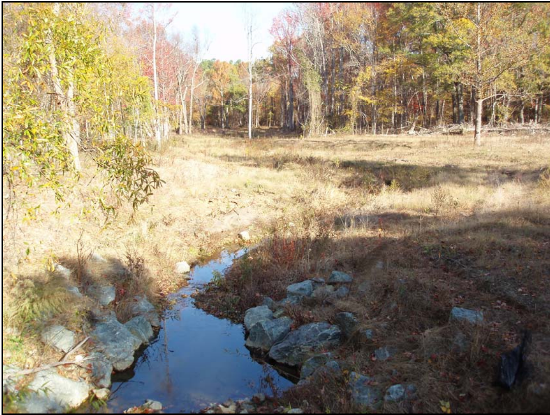
Photo Point 6: View looking north from Gerring Road culvert. 11/16/07 – MY-01
