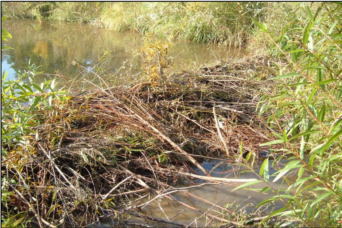
Beaver Dam – First of two beaver dams at the site. Station 19+50 09/29/08 - MY 02
