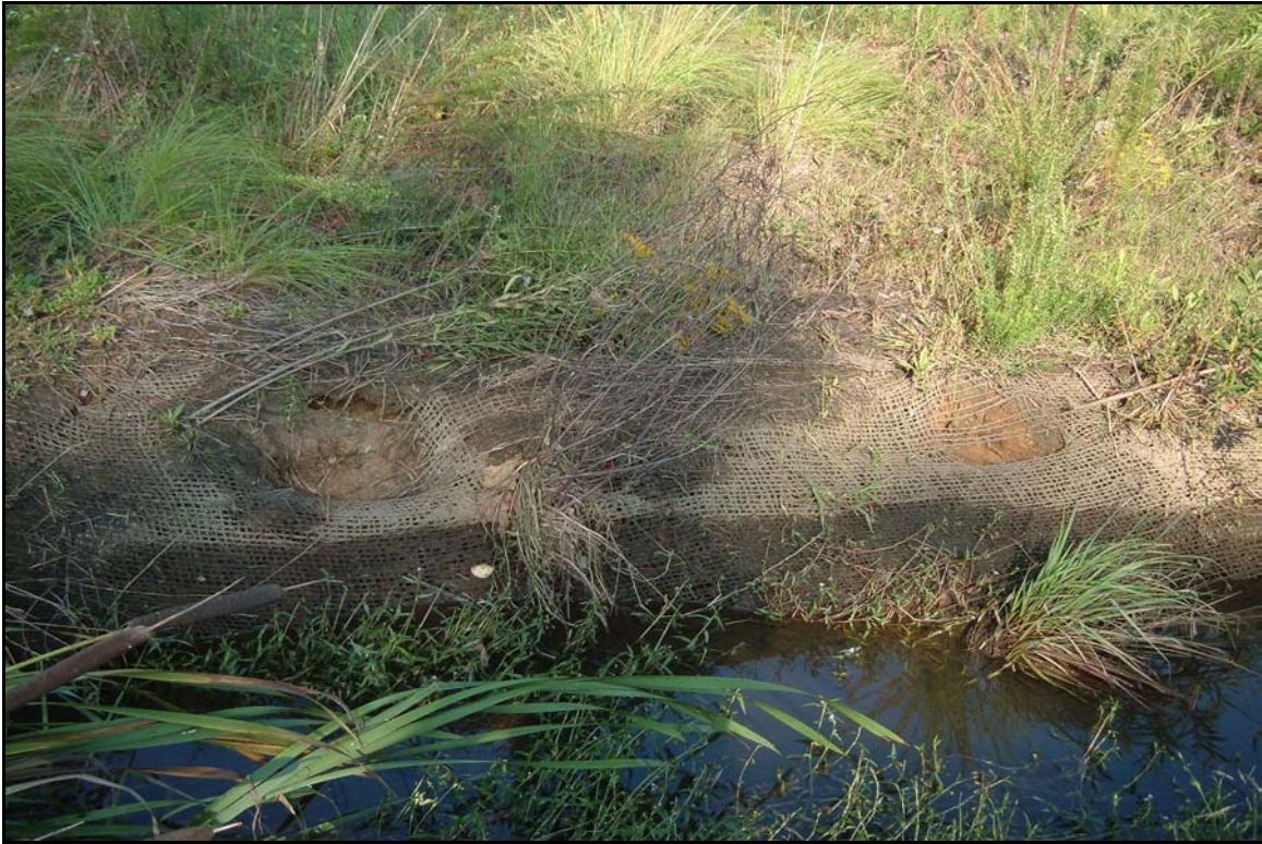
Bank Erosion – Erosion on toe of bank beneath matting. Stationing 11+10 – 11+25 09/29/08 - MY 02
