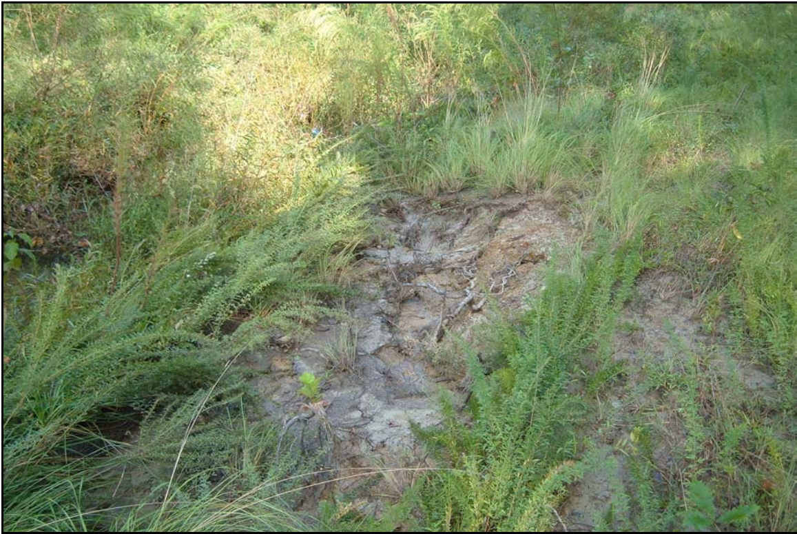
Floodplain Erosion – Upper bank and floodplain erosion. Stationing 31+85 – 32+05 09/29/08 - MY 02
