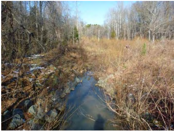
Photo Point 6: View looking north from Gerring Road culvert. 12/10/10 – MY-04
