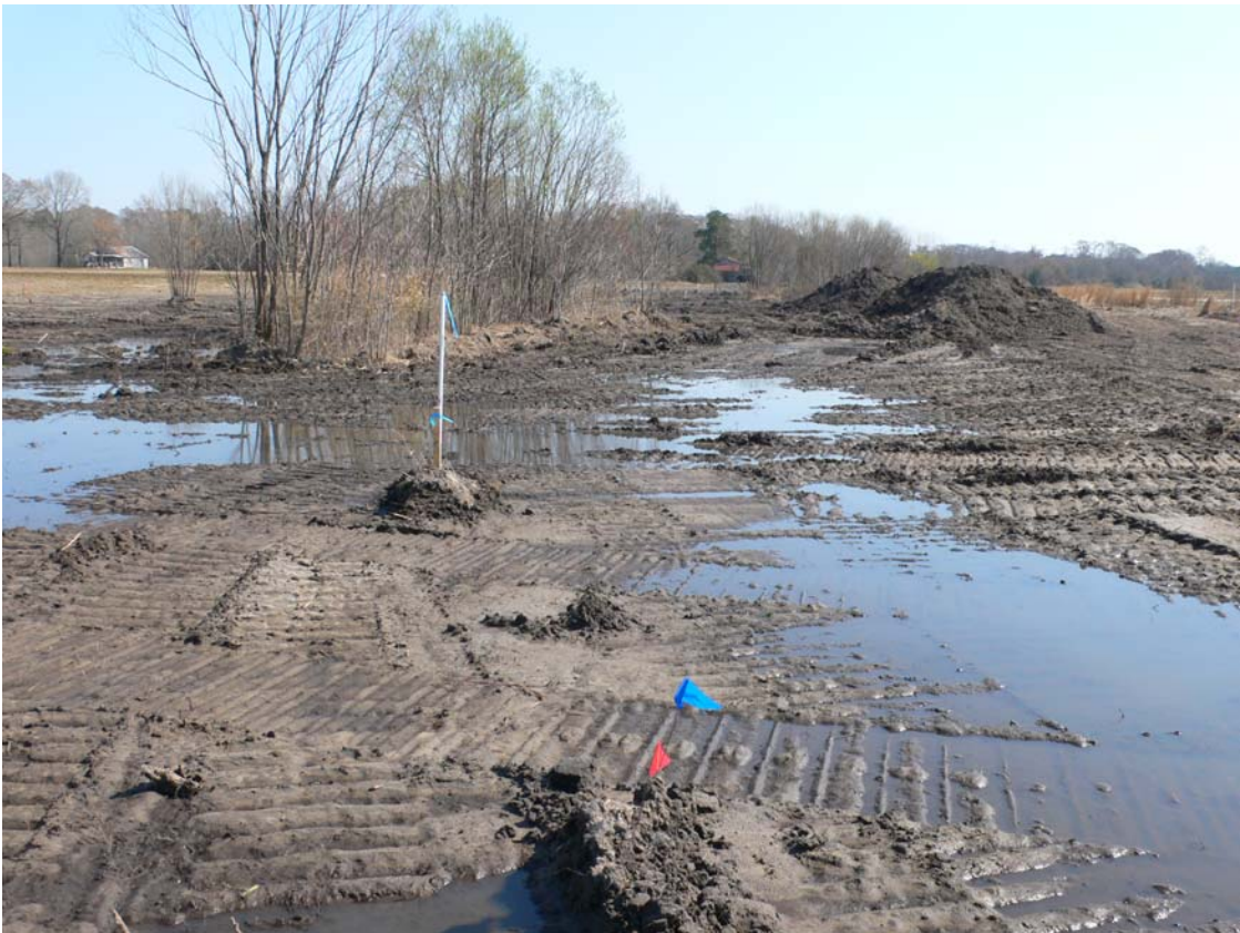
Photo 7: Initial cutting and stockpiling of topsoil.
