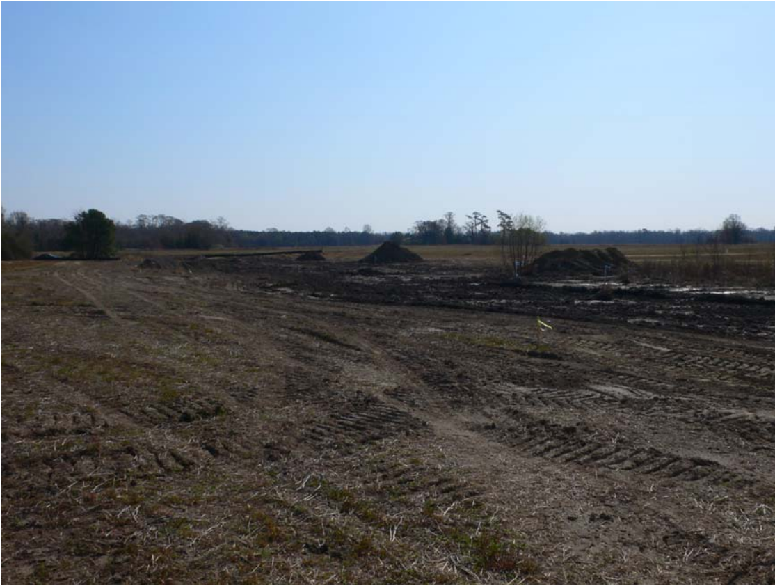
Photo 5: Swamp run grading and stockpiling of topsoil.
