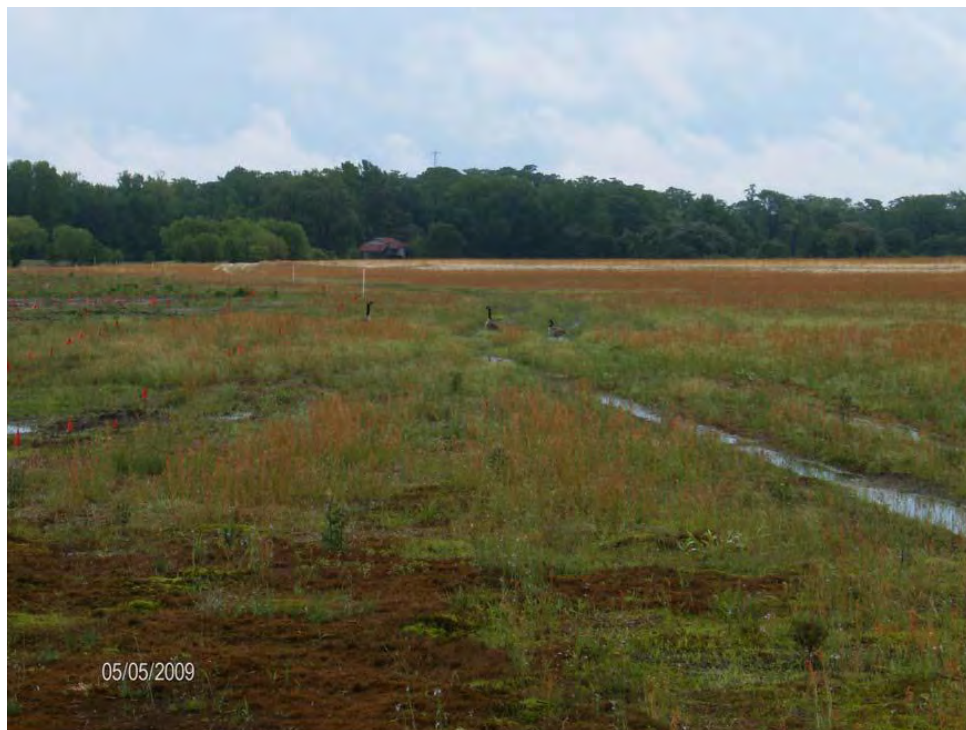
Looking downstream in the northern restored swamp run one month post-construction.
