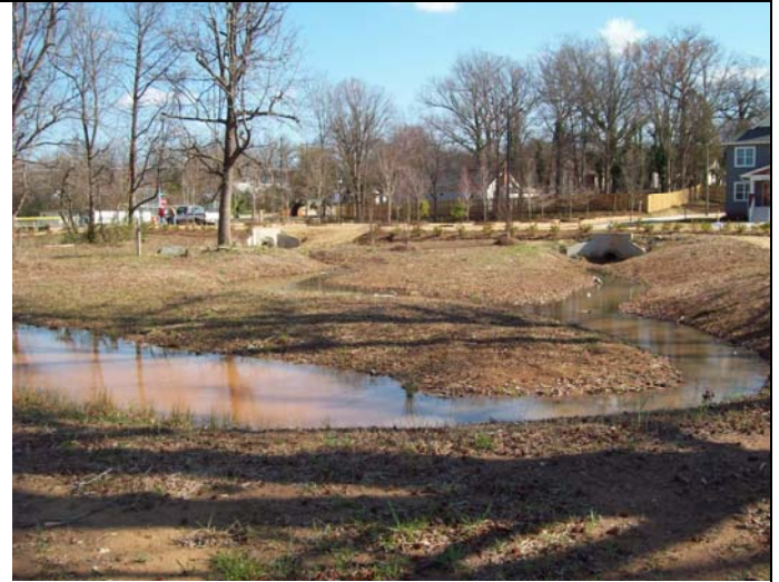
Eastway reach, stormwater channels, ~ sta. 2+00.
