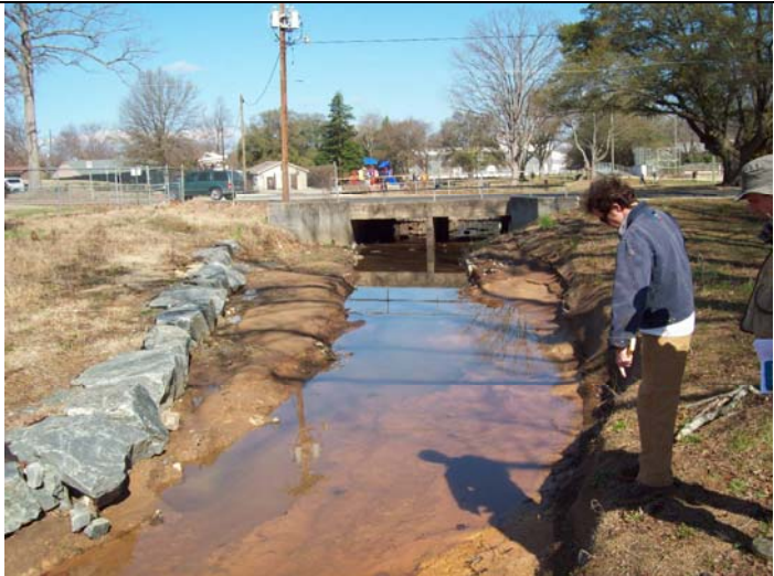
Eastway reach, looking downstream, ~sta.1+00.
