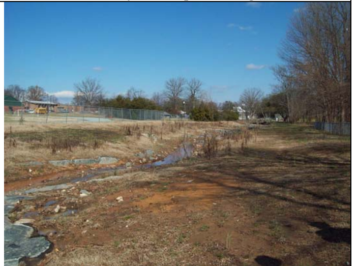
Eastway reach, right bank looking downstream, ~ sta. 6+00.
