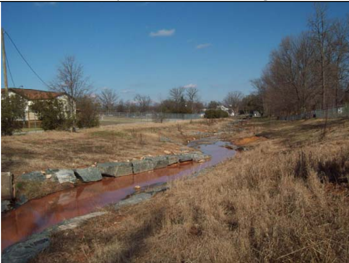
Eastway reach, upstream, right bank, looking downstream, ~ sta. 8+00.
