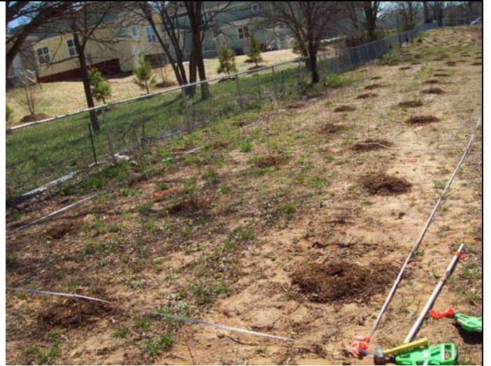
Plot 4, Eastway reach, upstream, right bank.
