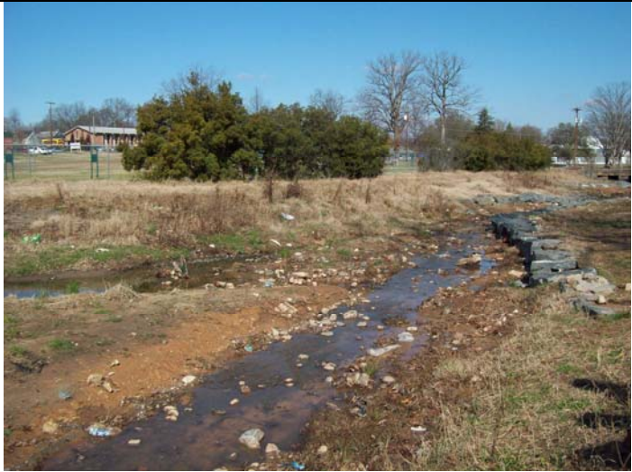
Eastway reach, looking downstream, ~ sta. 3+00.
