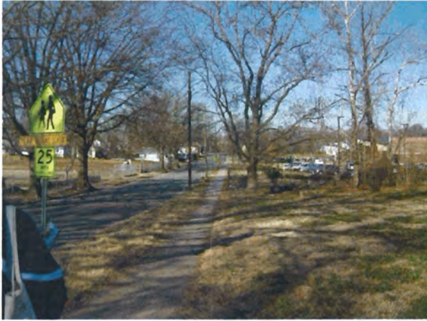
Photograph 1. Looking west along Taylor Street towards Eastway Elementary School. Goose Creek contained in culvert from this location upstream to Upper Reach (1/21/04).
