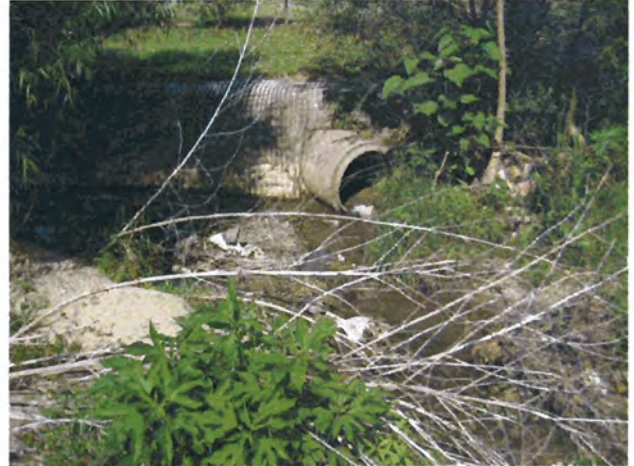
Photograph 14. Looking at outfall draining into reach. (5123105)
