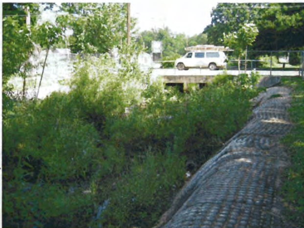
Photograph 17. Looking downstream at culvert under Liberty Street, spring foliage. (5123105)
