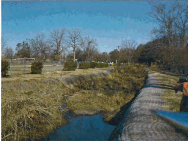
Photograph 13. Looking downstream along exposed grouted mattress lining covering right bank. (1/21/04)
