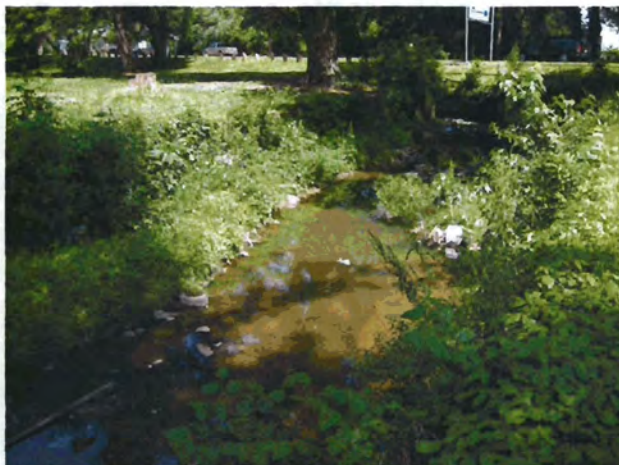
Photograph 23. Looking downstream at Holloway Street culvert, downstream reach limit. (5/23/05)
