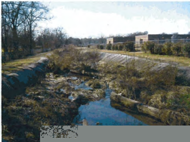
Photograph 15. View upstream from lower portion of reach with log deflectors visible. (1/21/04)
