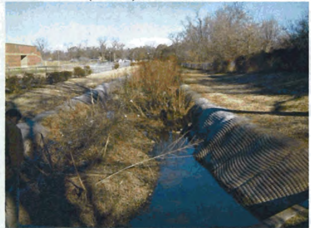
Photograph 4. Looking downstream from Taylor Street outfall, with winter foliage. (1121104)
