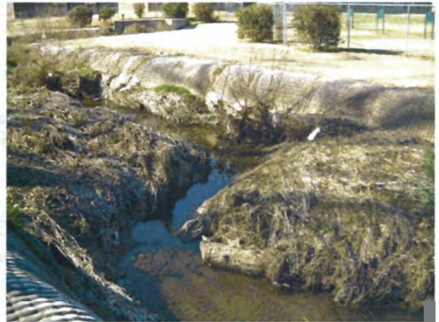
Photograph 12. Looking upstream at meandering low flow channel midreach. (1/21/04)
