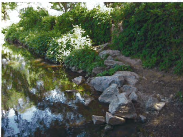
Photograph 17. Looking downstream along arm of rock vane structure. (5/23/05)
