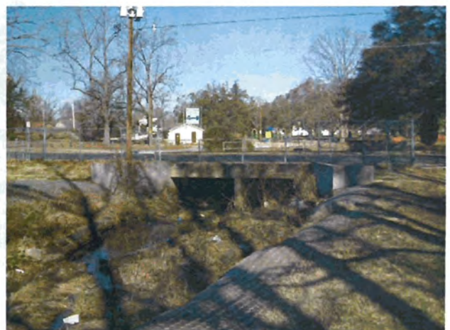
Photograph 18. Looking downstream at Liberty Street culvert, winter foliage, downstream reach limit. (1121104)
