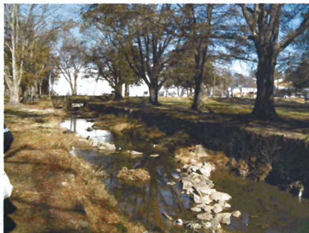
Photograph 16. Looking downstream towards culvert under Holloway Street. (11/21/04)
