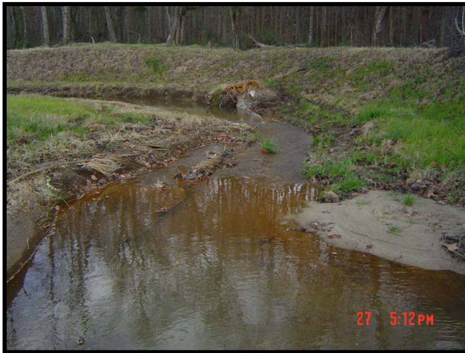
Typical Bank Scour—Reach —Year 1 (2006)
