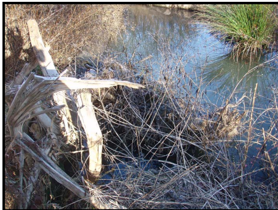
Typical Stressed Structure/Bank Scour—Reach 1—Year 2 (2007)
