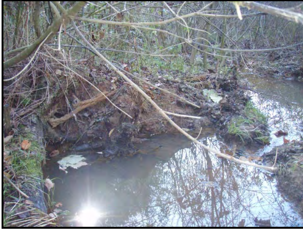
Photo 5 – Typical Stressed Structure/Bank Scour – Reach 2 – Year 5 (2010)
