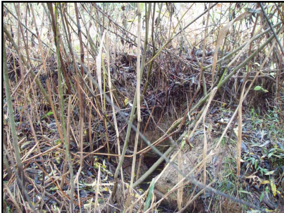
Photo 2 – Typical Stressed Structure/Bank Scour – Reach 1 – Year 5 (2010)
