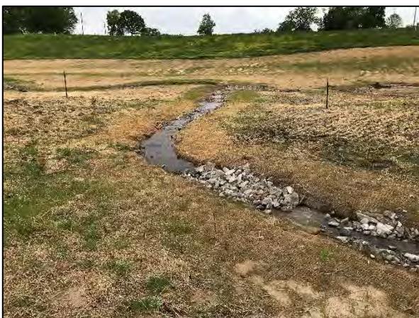
Photo Point 16 – UT1A, Sta. 12+00 Facing Downstream (4/29/2020)
