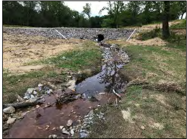
Photo Point 4 – UT1 Reach 1, Sta. 15+00 Facing Downstream (4/29/2020)
