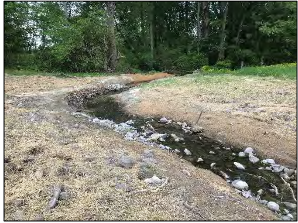
Photo Point 14 – UT1 Reach 3, Sta. 29+45 Facing Downstream (4/29/2020)
