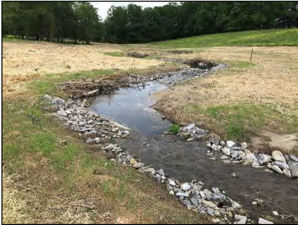
Photo Point 9 – UT1 Reach 3, Sta. 22+40 Facing Downstream (4/29/2020)
