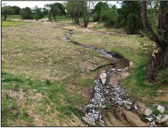
Photo Point 1 – UT1 Reach 1, Sta. 10+00 Facing Downstream (4/29/2020)
