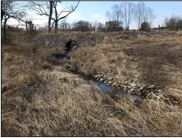
Photo Point 17 – UT1 Reach 1, Sta. 16+50 Facing Upstream (2/10/2021)
