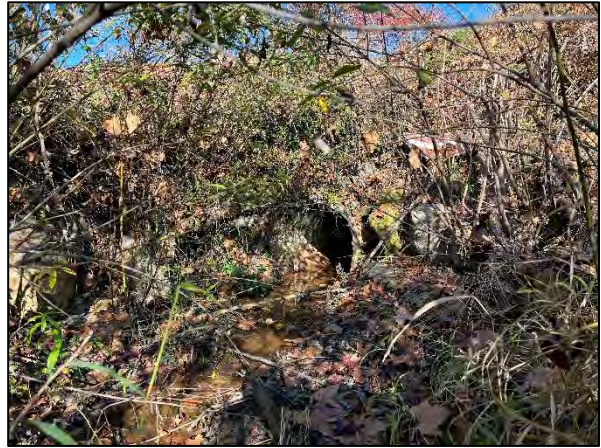
Photo Point 18 – UT1 Reach 1, Sta. 10+30 Facing Upstream (11/3/2022)
