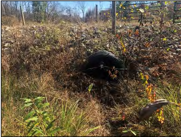
Photo Point 19 – UT1 Reach 1, Sta. 15+50 Facing Downstream (11/10/2022)
