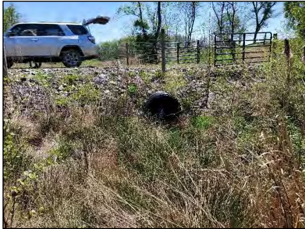
Photo Point 19 – UT1 Reach 1, Sta. 15+50 Facing Downstream (04/11/2023)
