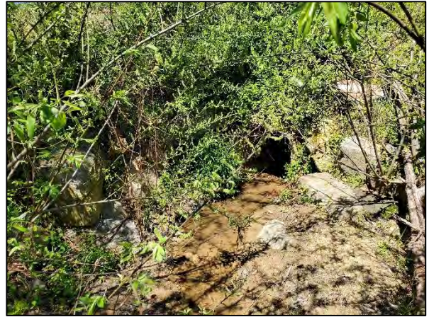
Photo Point 18 – UT1 Reach 1, Sta. 10+30 Facing Upstream (4/11/2023)
