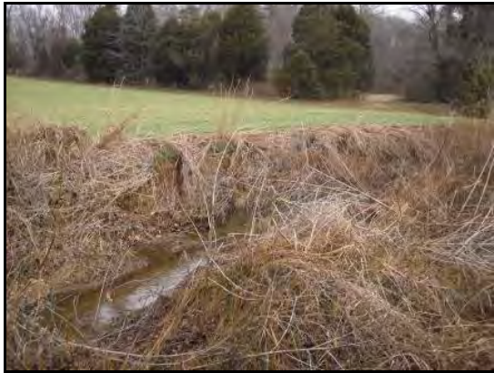
UT1: Facing upstream showing absent riparian buffer.
