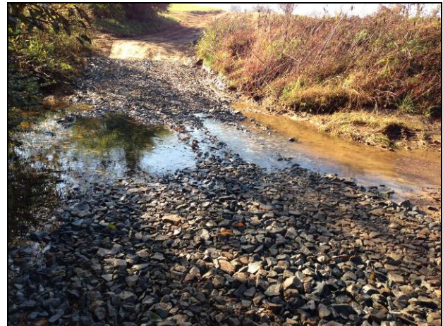
Photo 17-UT1-Forward Stream Crossing after stabilization (November 2012).
