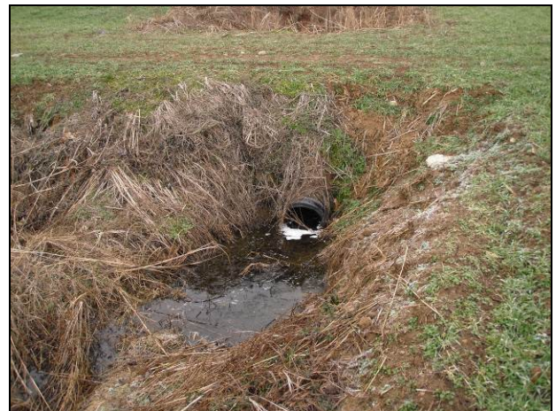
Photo 18-UT3-Stream Crossing pre-stabilization (January 2011).
