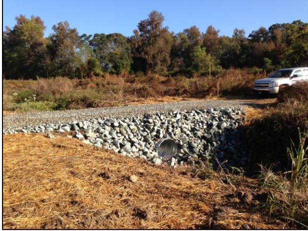
Photo 19- UT3-Stream Crossing after stabilization (November 2012).
