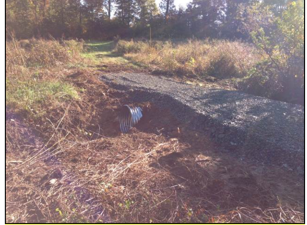
Photo 21- UT4-Stream Crossing after stabilization (November 2012).
