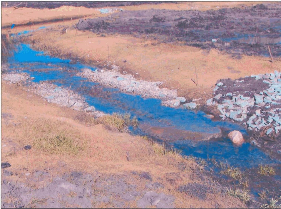
Photo P4. A constructed riffle near the end of Reach 1.
