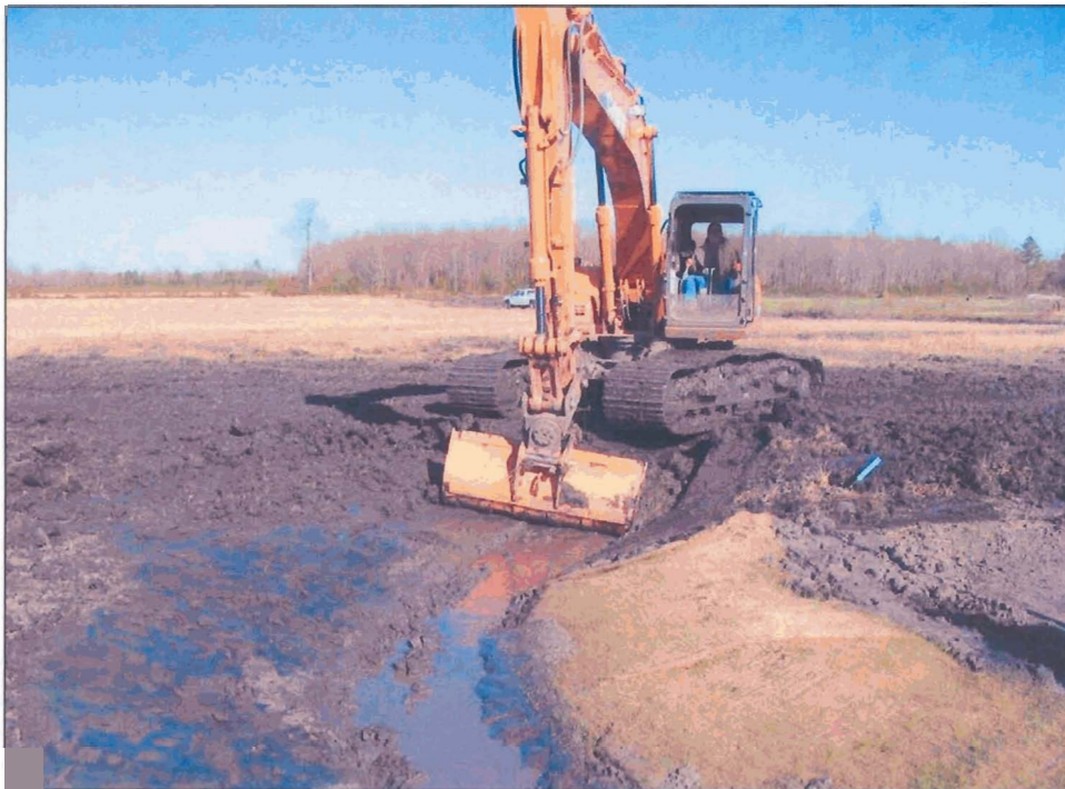
Photo C2. A new section of stream channel (Reach 2) during excavation.
