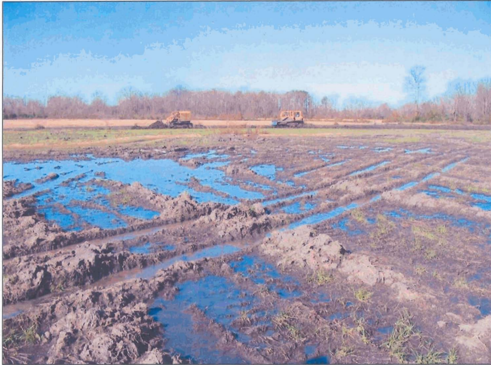
Photo C1. Restoration area during initial grading to design elevations.
