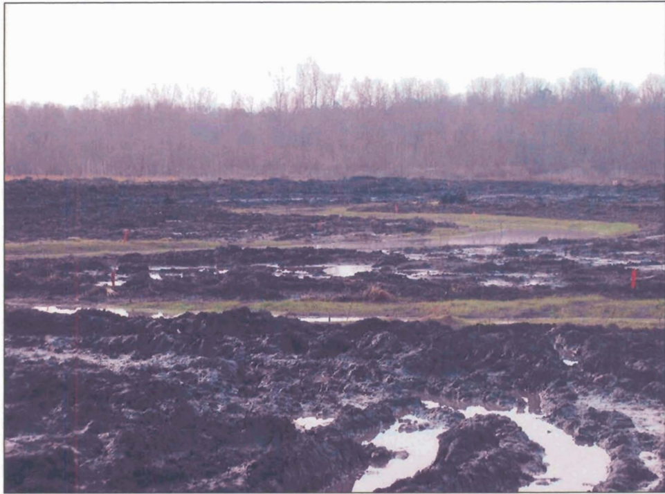
Photo P5. Middle portion of the project. Scarification and minor grading resulted in a diversity of hydrologic wetland conditions.
