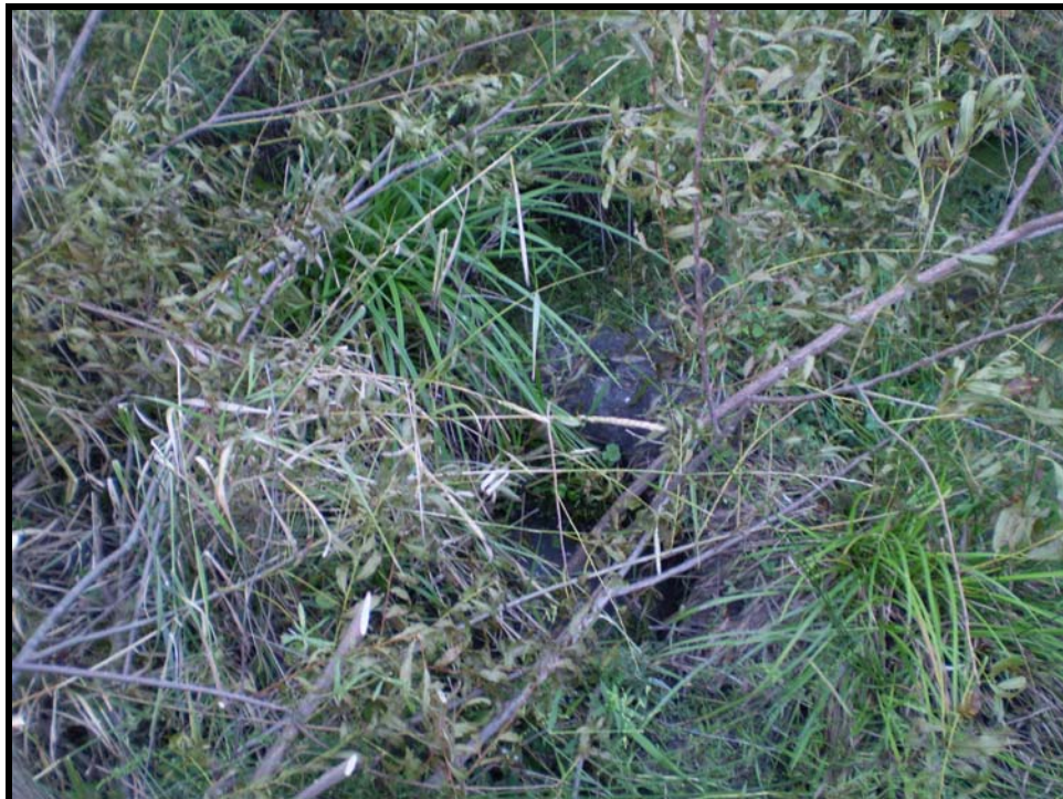
SPA 2. Right bank erosion at station 41+00.
