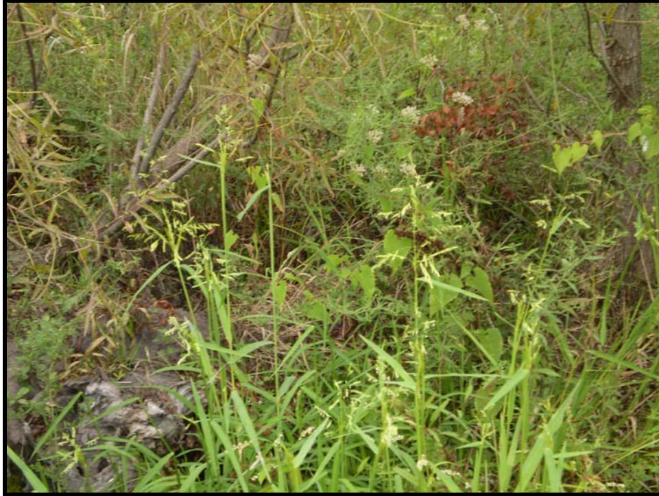
SPA 3. Erosion behind root wad at station 42+00.
