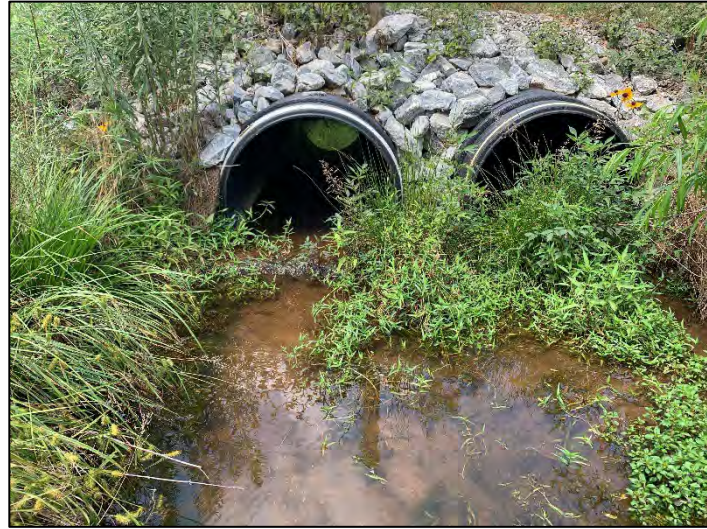
Crossing GF1-B – Upstream (7/5/2022)
