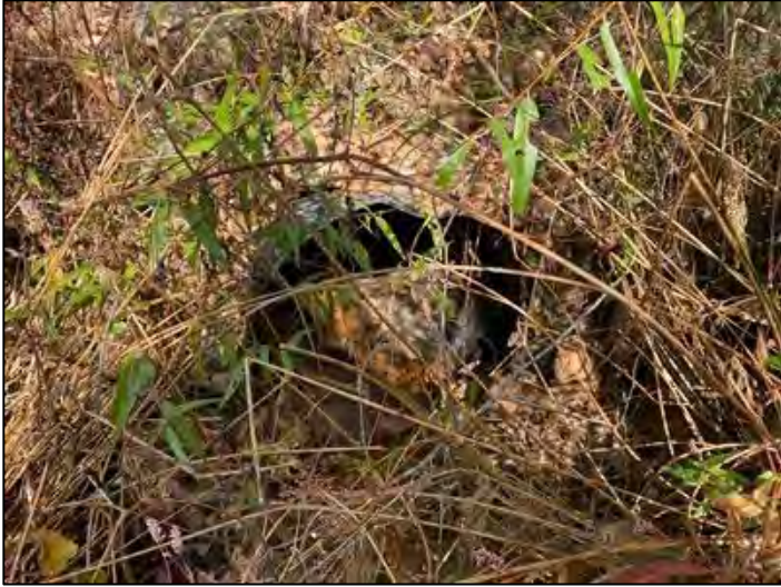
GF4A Crossing - Downstream
