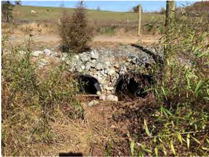
Crossing GF3 – Downstream (10/25/2022)
