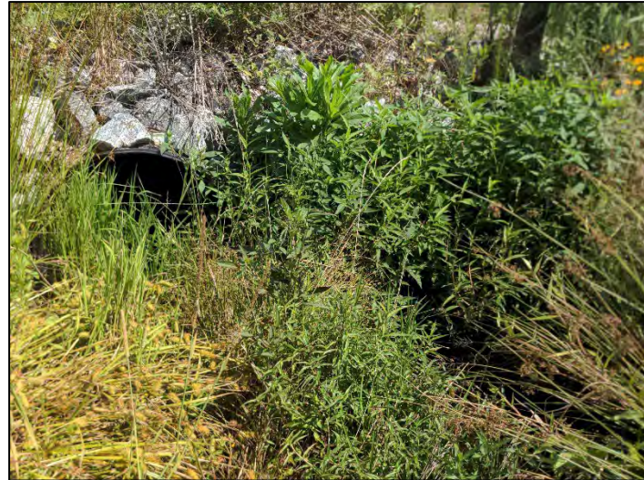
Crossing GF2-B – Downstream (7/5/2022)
