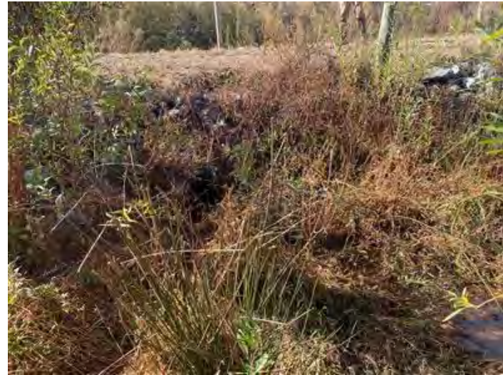
Crossing GF3 – Upstream (10/25/2022)
