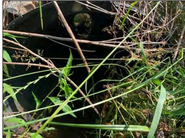
Crossing GF2-B – Downstream
