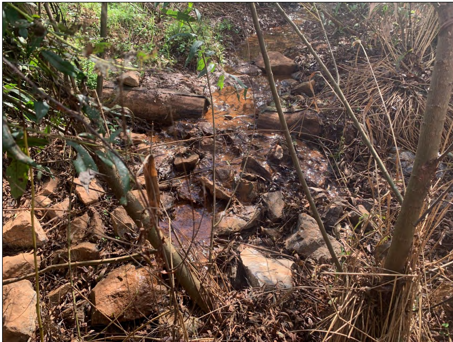
GF4 Structure Repair (looking Upstream)
