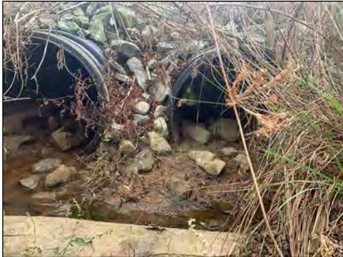
Crossing GF2-B - Upstream
