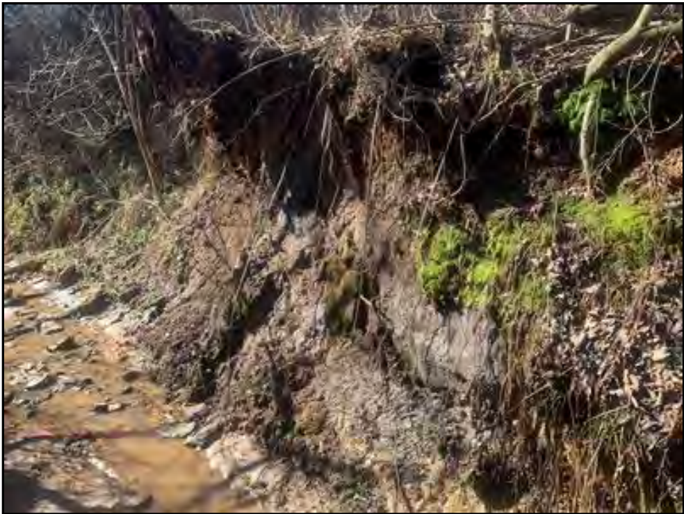
Eroding Slope – GF3A (02/13/2024)
