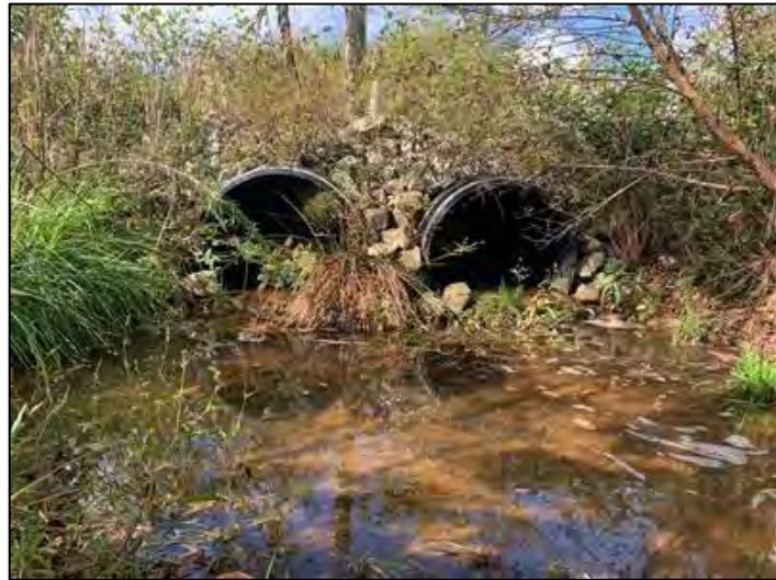
Crossing GF1-B – Upstream
