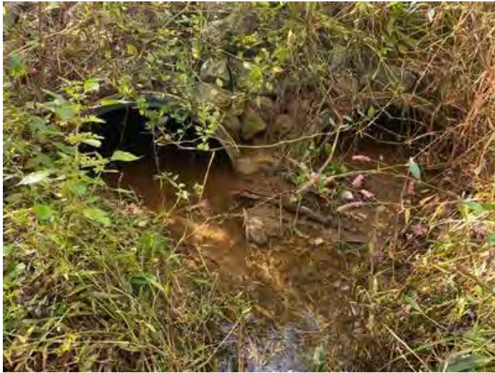
Crossing GF3 – Downstream)
