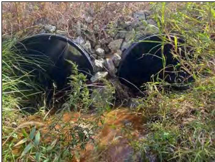
Crossing GF1-B – Downstream
