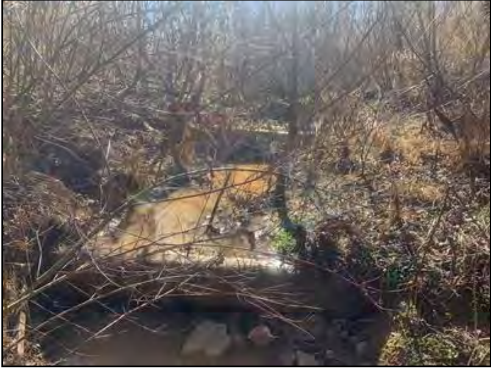
Log Sills GF3-A (02/13/2024)
