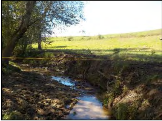
Reach GF1-B – Middle Looking upstream
