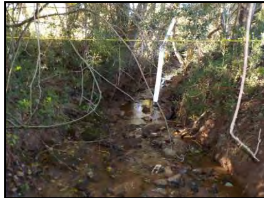
Reach GF3-A – Looking downstream
