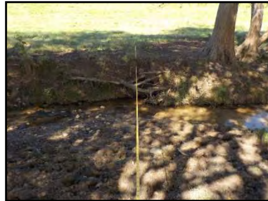
Reach GF1-B – Middle Looking at left bank
