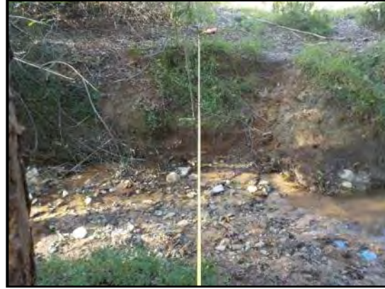
Reach GF2-B – Looking at left bank
