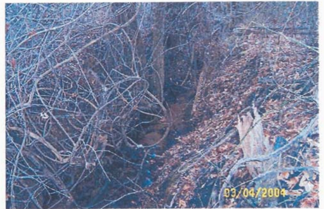
On-Site Pool Cross-section 4 looking upstream
