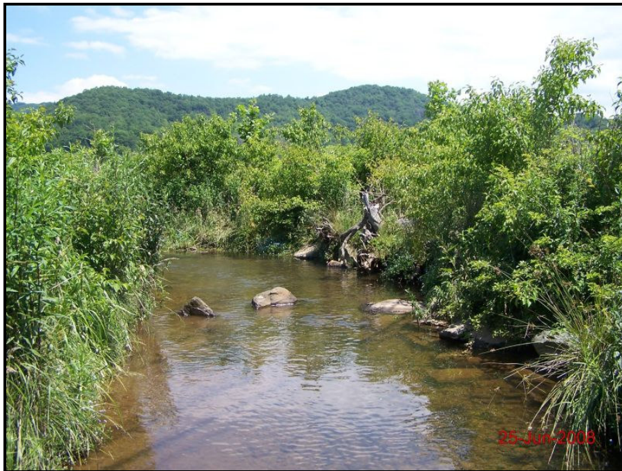
Stream Problem Area (SPA 4) – Failed engineered structure Monitoring Year 5 – June 25, 2008
