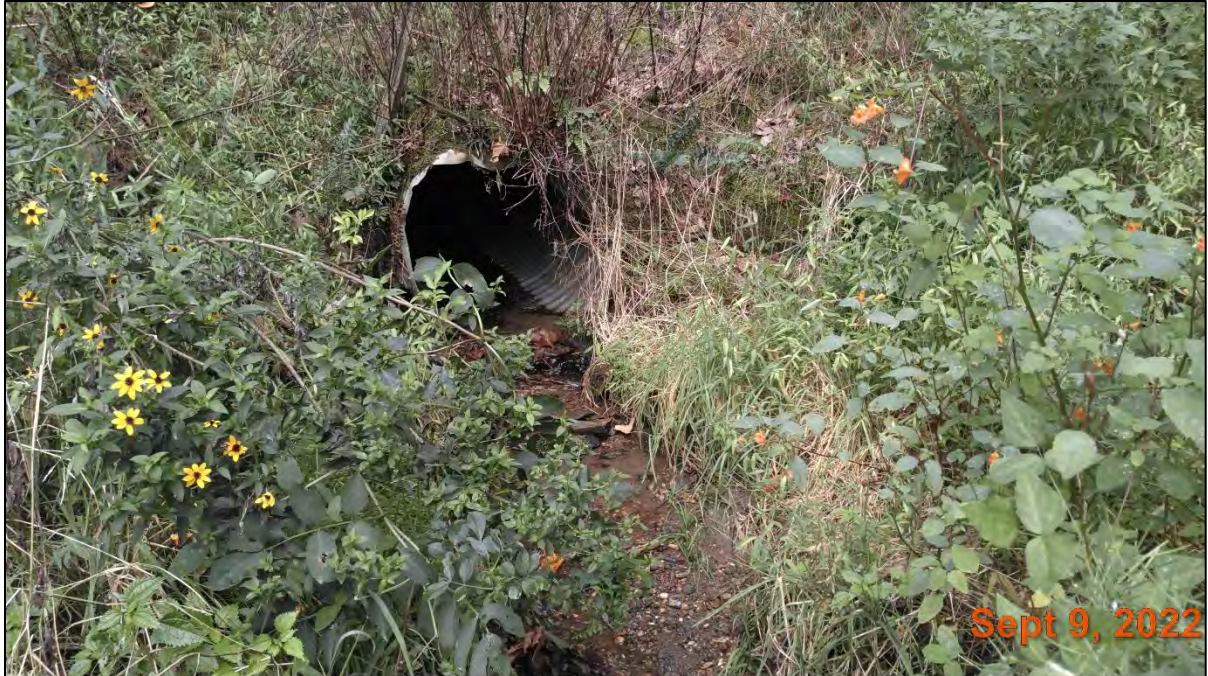
Photo point #1e facing upstream at Reach 1A/B culvert.
