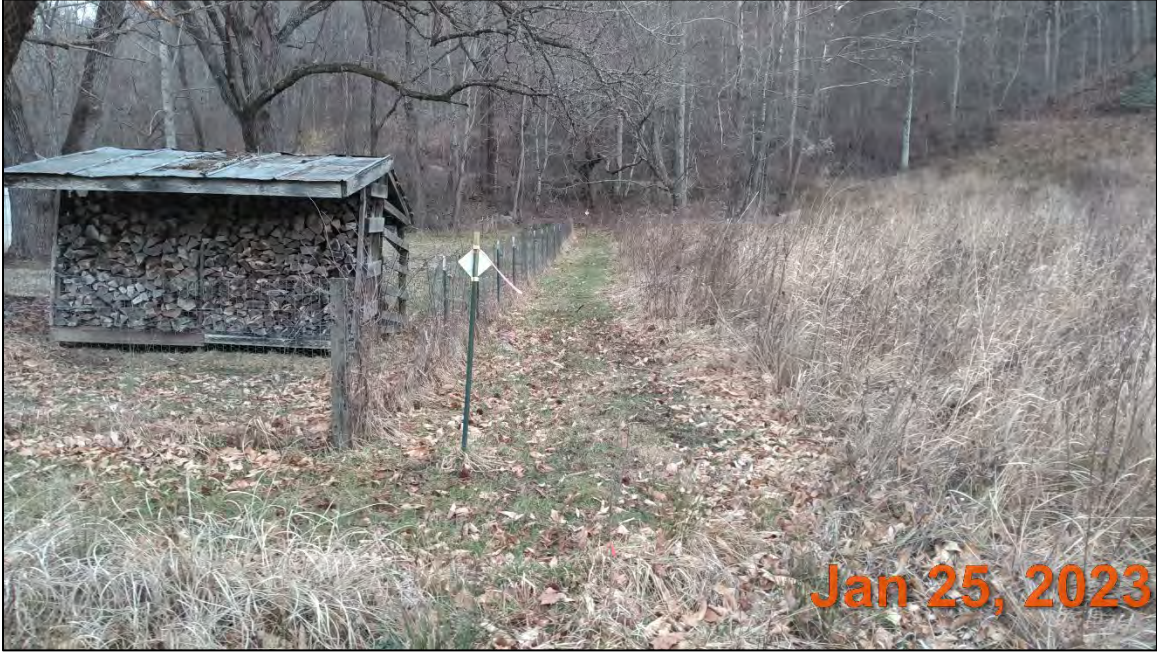
Easement Violation (Mowing) along residential fence line.
