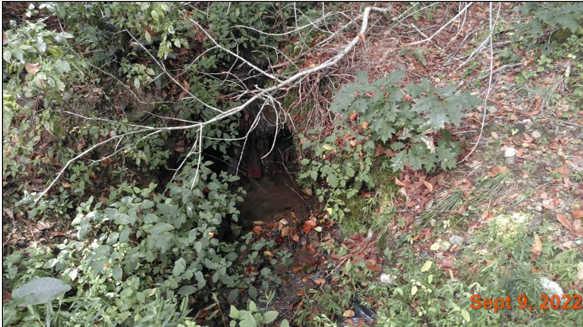
Photo point #1b, facing stormwater control measure along Reach 1A boundary.
