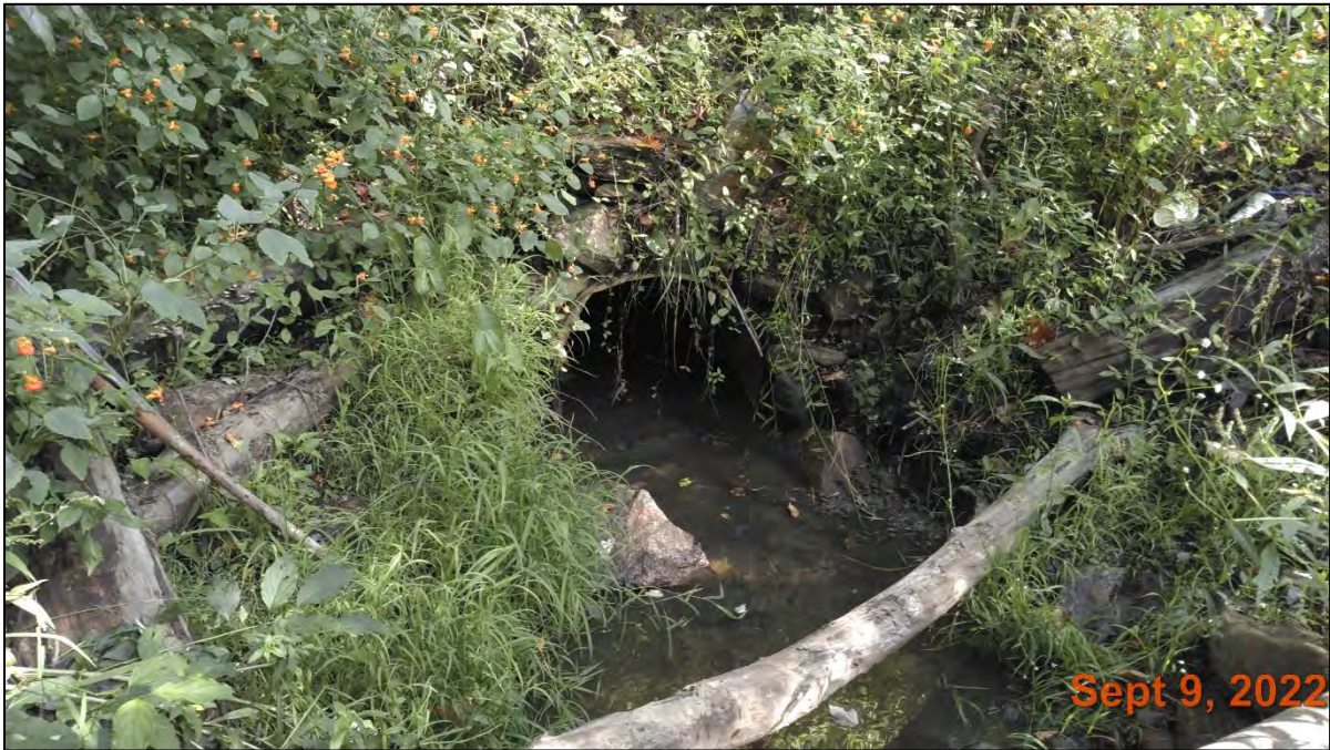
Photo point #8b, facing downstream Caney Fork Road culvert, Reach 1D.
