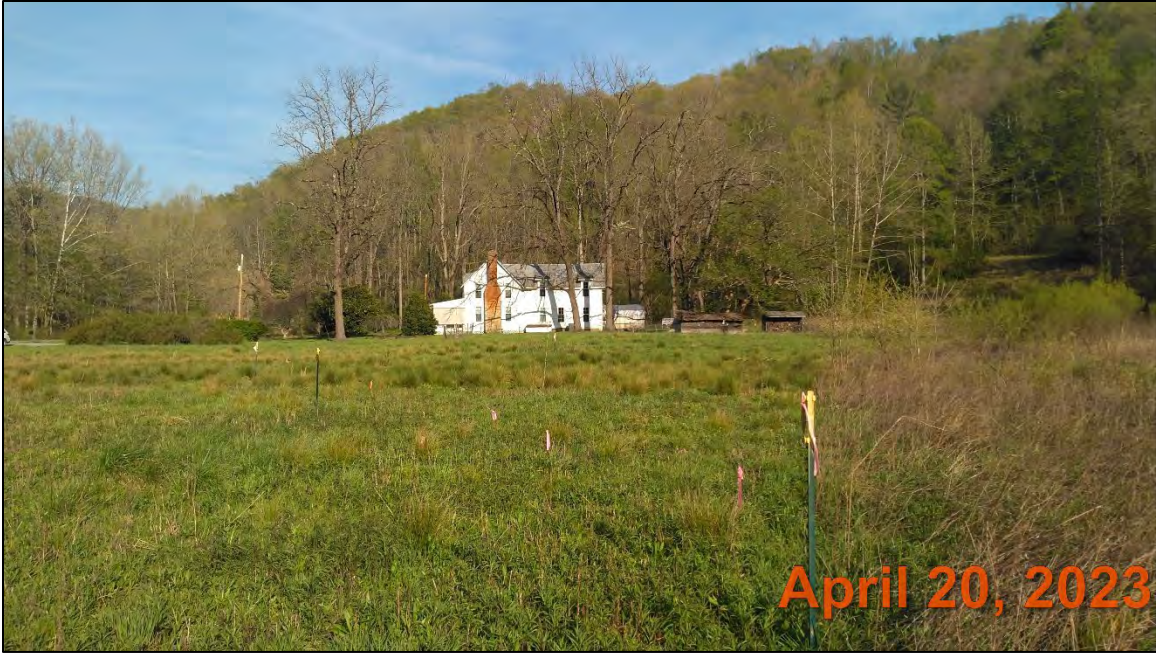
Replanted Easement Violation (Mowing) Station 103+00 to 105+50
