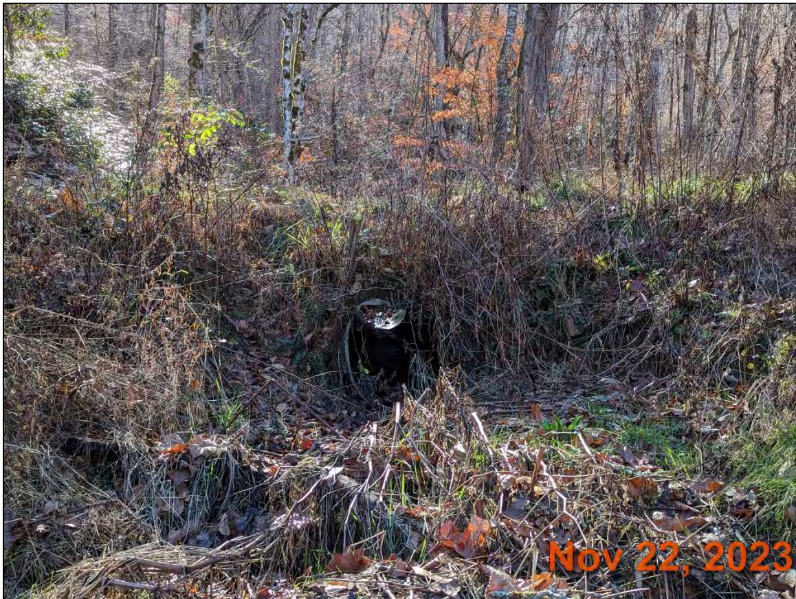
Photo point #1f facing upstream through the Reach 1A/B culvert.
