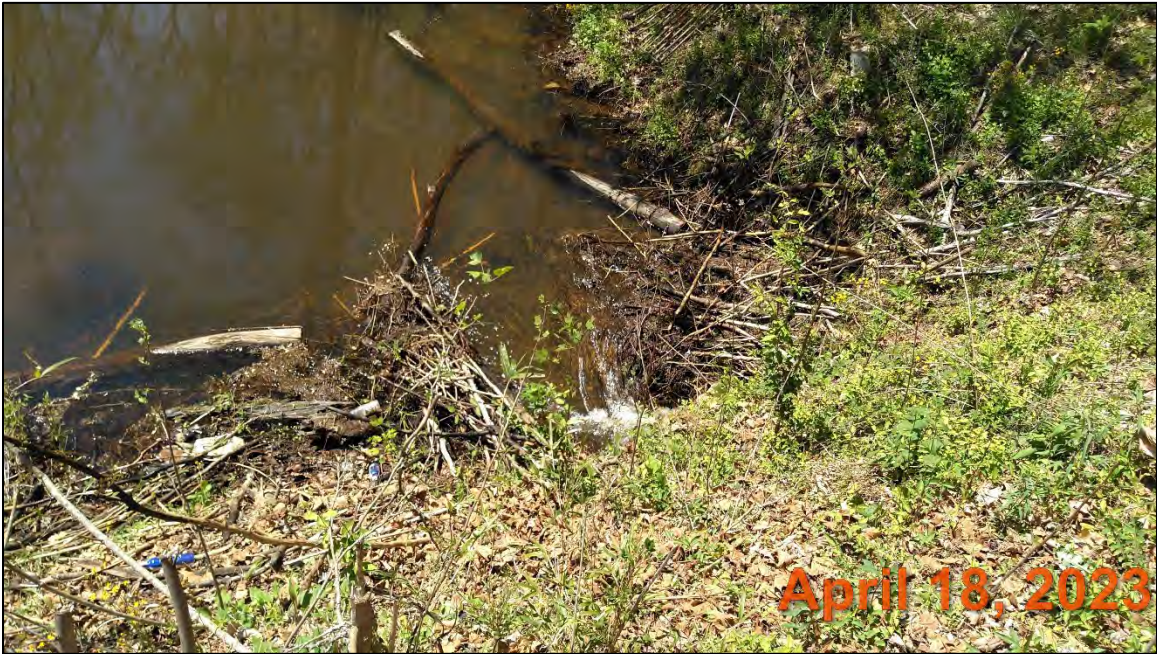
Beaverdam at Caney Fork Rd Culvert
