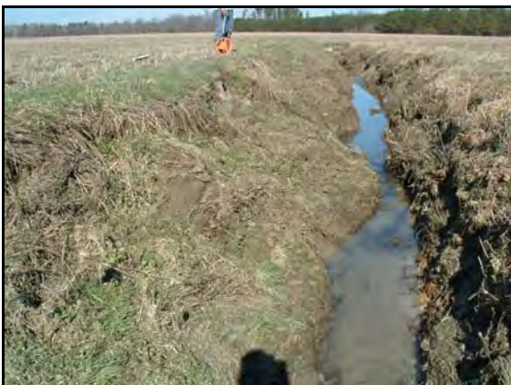
Eroding banks along the project stream.
