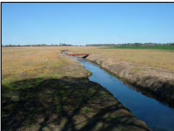
Looking upstream from the end of the project stream.
