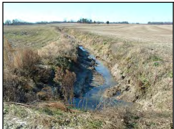
Looking upstream from the second road crossing.
