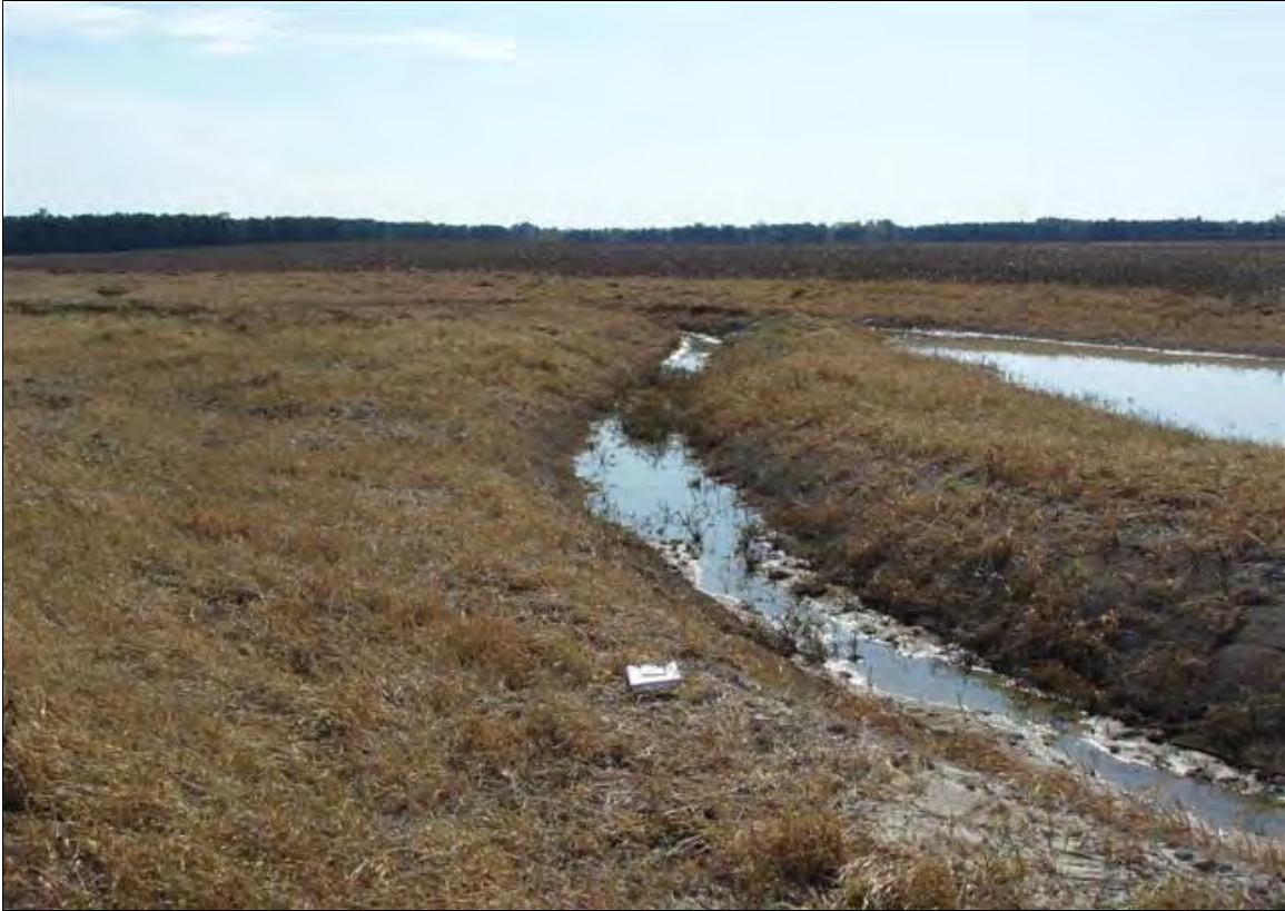
Photo Point S13: View looking downstream near Station 61+50. 11/7/07 – As-Built
