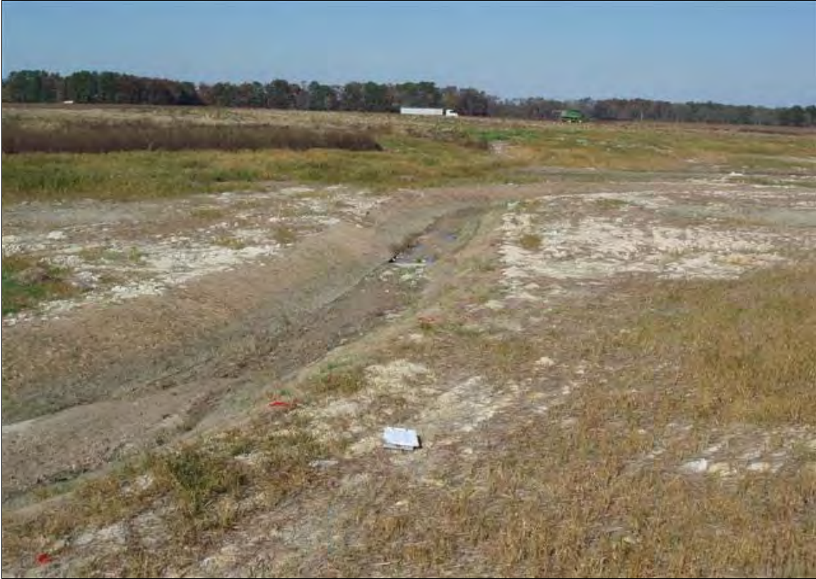
Photo Point S7: View looking downstream near Station 39+00. 11/7/07 – As-Built
