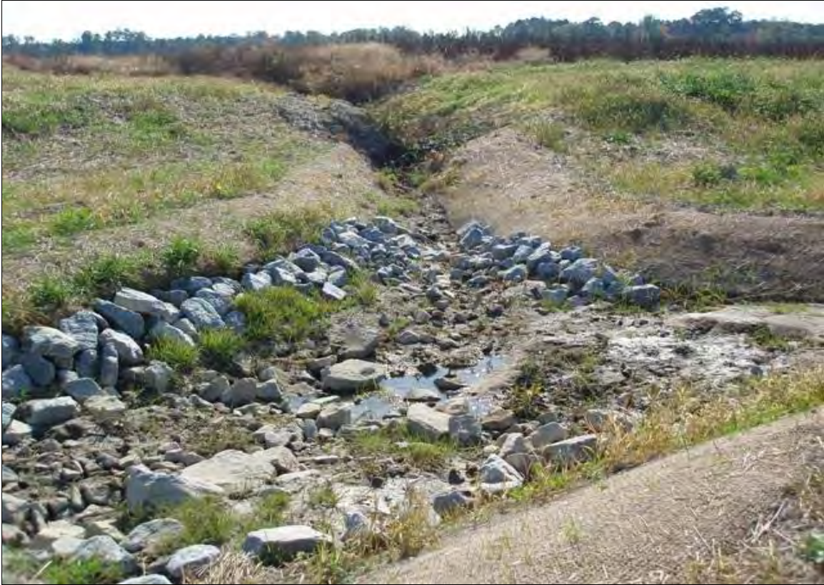
Photo Point S6: View of drainage ditch reinforcement, near Station 37+25. 11/7/07 – As-Built
