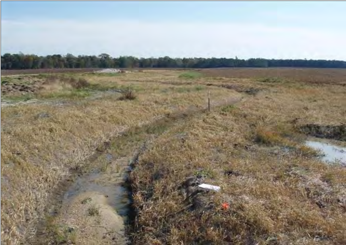
Photo Point S12: View looking downstream near Station 52+00. 11/7/07 – As-Built
