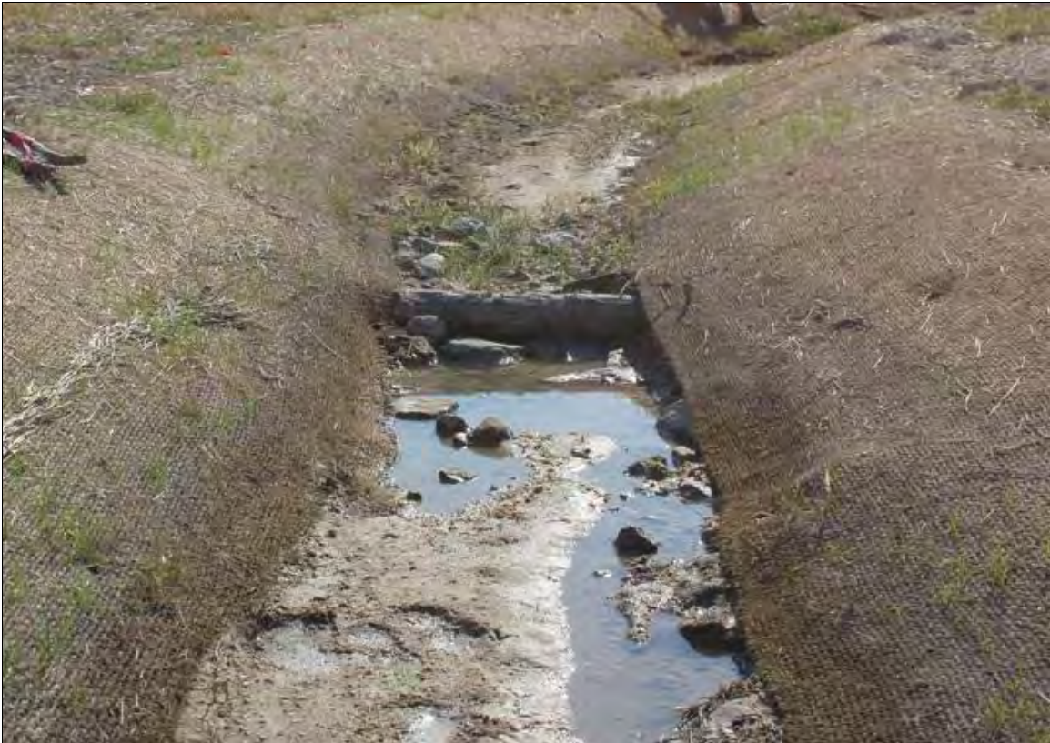
Photo Point S8: View of log drop structure near Station 39+50. 11/7/07 – As-Built
