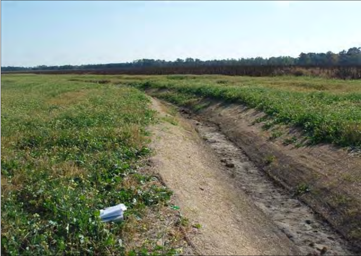
Point S3: View looking downstream near Station 27+60. 11/7/07 – As-Built
