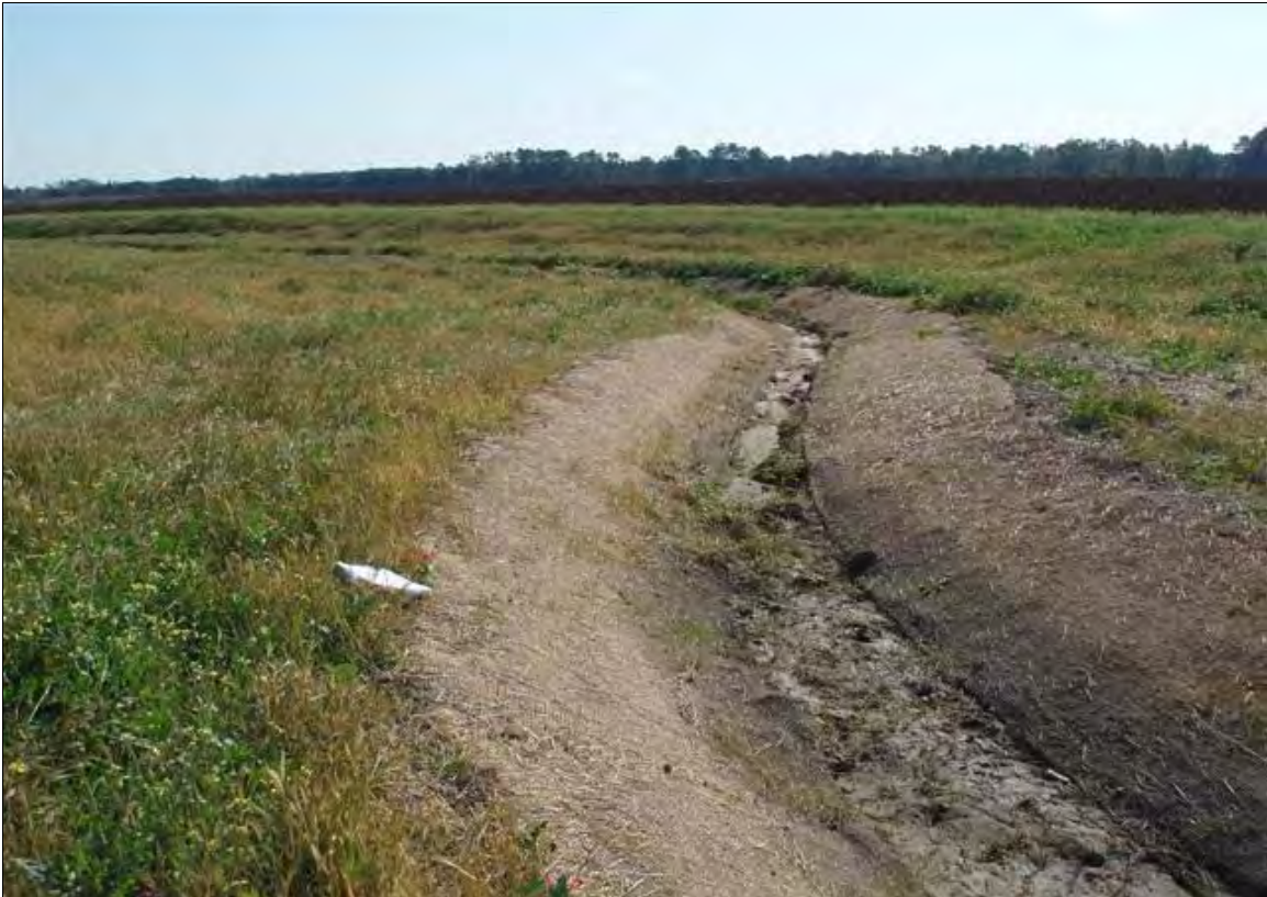
Photo Point S5: View looking downstream near Station 33+35. 11/7/07 – As-Built
