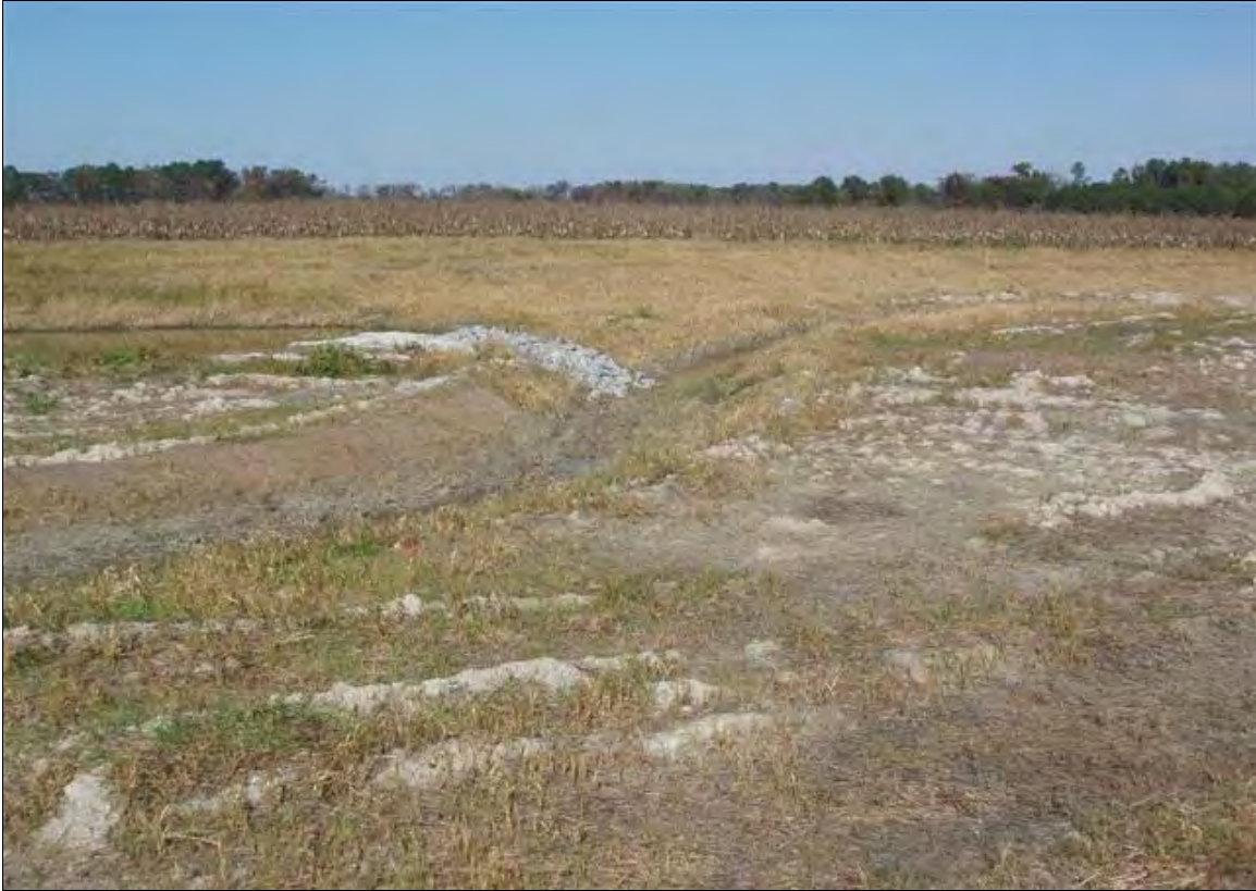
Photo Point S10: View looking downstream near Station 46+15. 11/7/07 – As-Built
