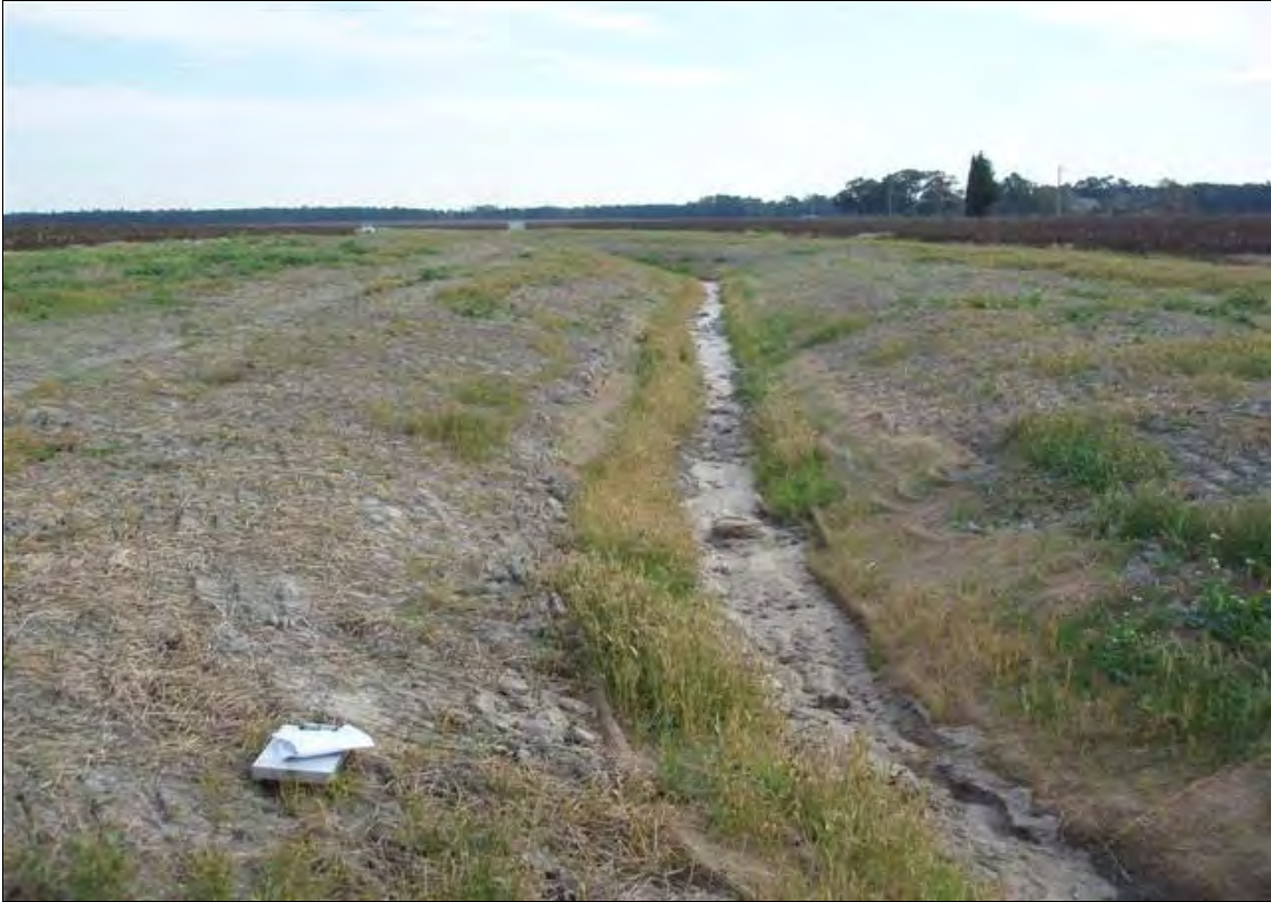
Photo Point S1: View looking downstream, near Station 12+75. 11/7/07 – As-Built
