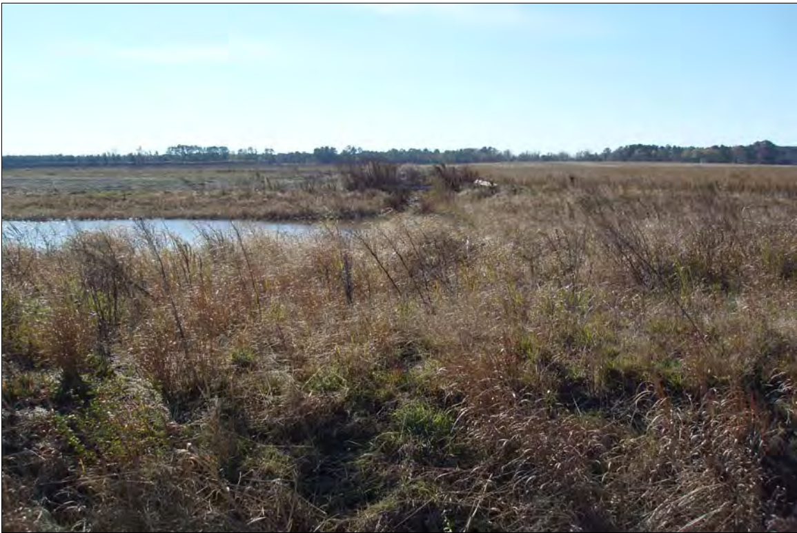
Photo Point S13: View of water quality treatment structure near Station 61+50. 11/19/08 - MY-01
