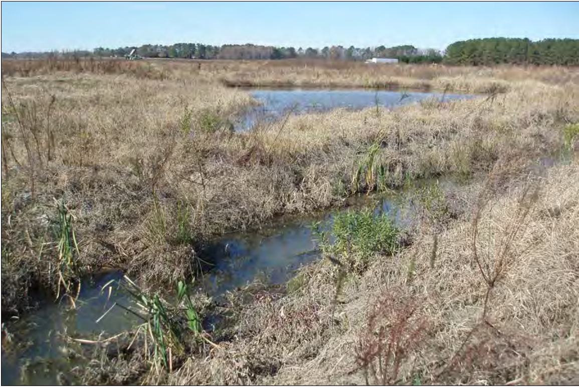
Photo Point S14: View of stream with water quality treatment structure in the background near Station 62+60. 11/19/08 - MY-01
