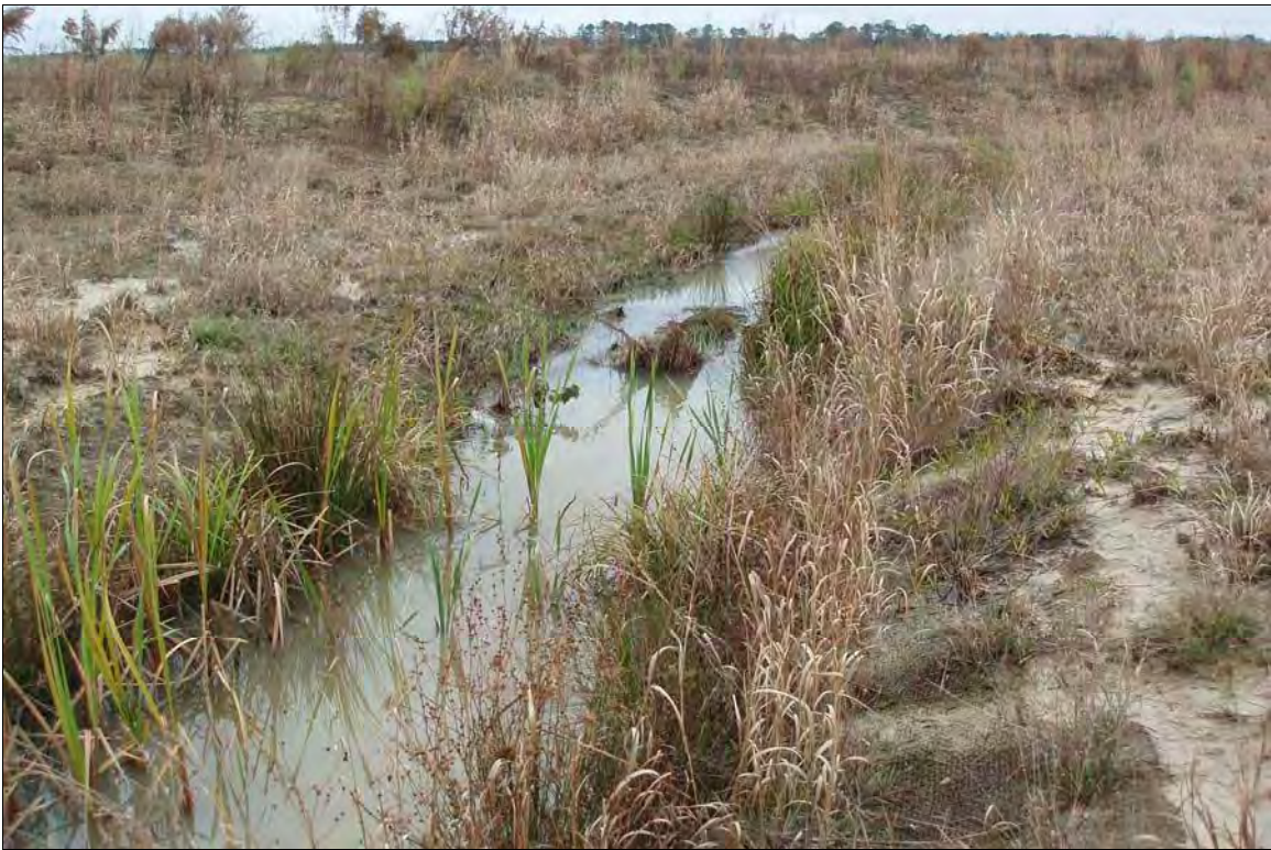
Photo Point S8: View of log drop structure near Station 39+50. 11/24/09 – MY-02
