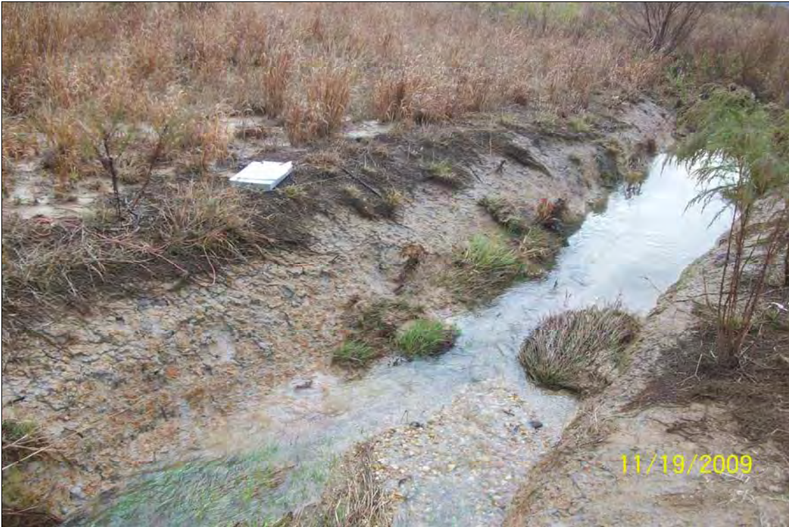
SP1 – Bed degradation near Station 33+40. 11/19/09 – MY-02
