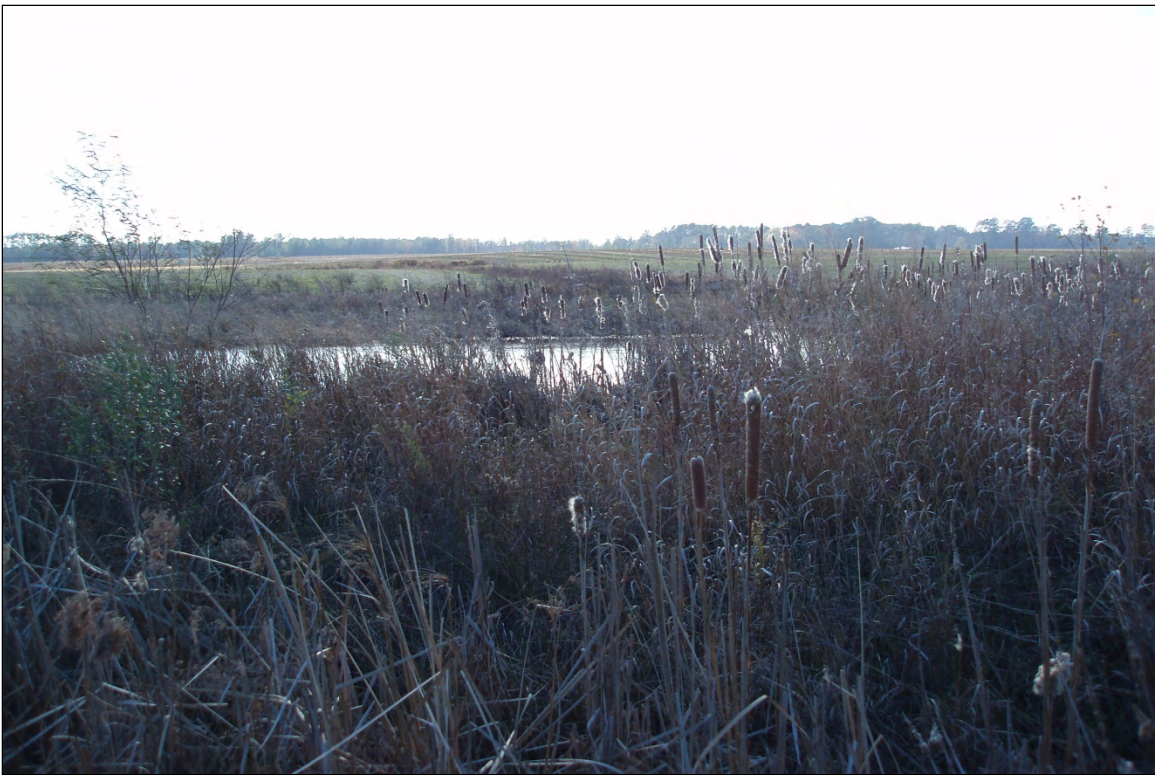
Photo Point S13: View of water quality treatment structure near Station 61+50. 12/6/10 – MY-03
