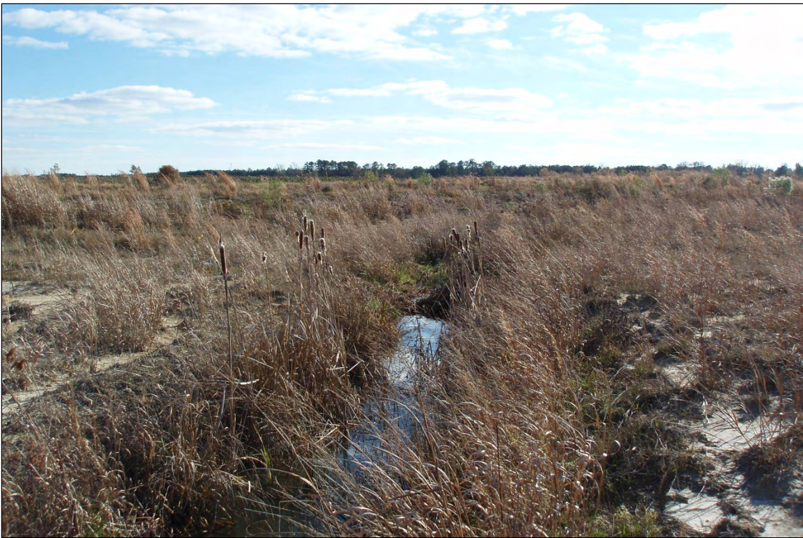
Photo Point S8: View of log drop structure near Station 39+50. 12/6/10 – MY-03
